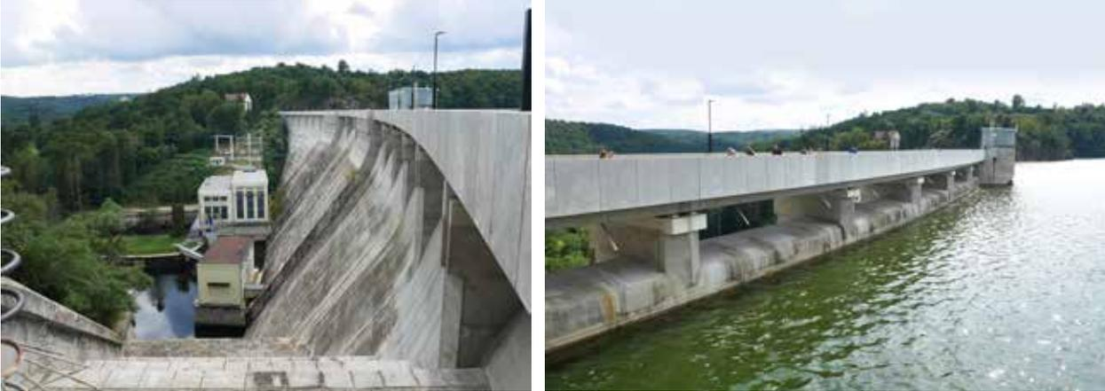
*Fig. 4.38: The Vranov dam (1930–1934) – example of a concrete dam and uncontrolled crown spillway (on the right). Photograph by Michaela Ryšková, 2020.*
