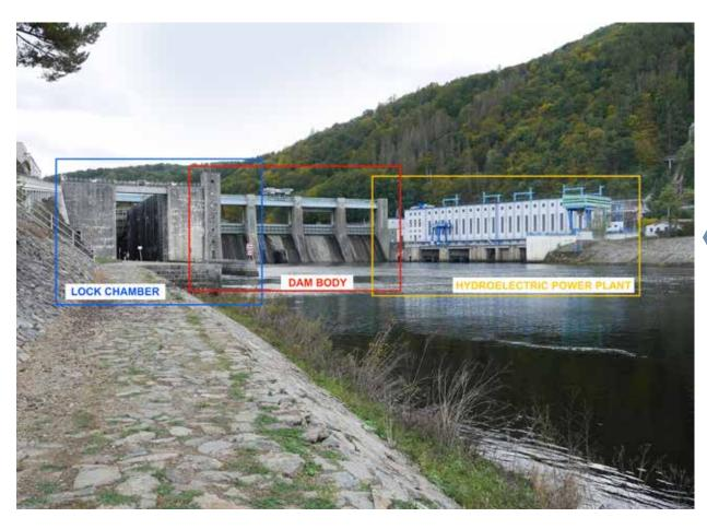
Fig. 4.59: The Štěchovice HS (1937–1945) – concrete gravity dam. Example of a functional complex – dam + lock chamber + hydroelectric power plant. Photograph by Michaela Ryšková, 2020.
