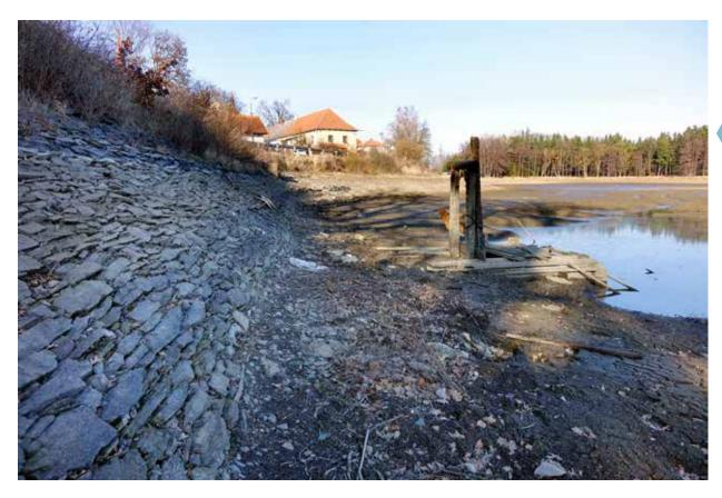
Fig. 4.77: Stone riprap of the upstream dam side of Zbýšovský Pond. Photograph by Jindřich Frajer, 2018.
