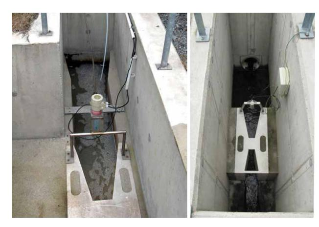
Fig. 4.279: The Purshall flume, an ultrasound sensor for the measurement of water flow (taken from: the TGM WRI archive).
