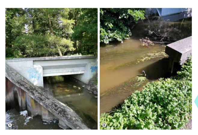
Fig. 4.116: The Semínský aqueduct on the Opatovice Canal. (A) state after reconstruction; (B) remains of old wooden elements. Photograph by David Honek, 2020.
