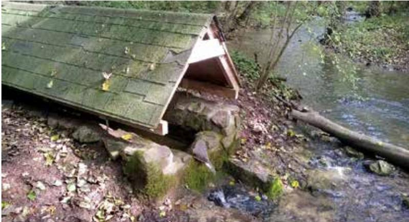
Fig. 4.231: Ochoz u Brna – spring tank (Kaprálůva studánka) catching underground water springs in close proximity to the Říčka River. Photograph by David Honek, 2014.
