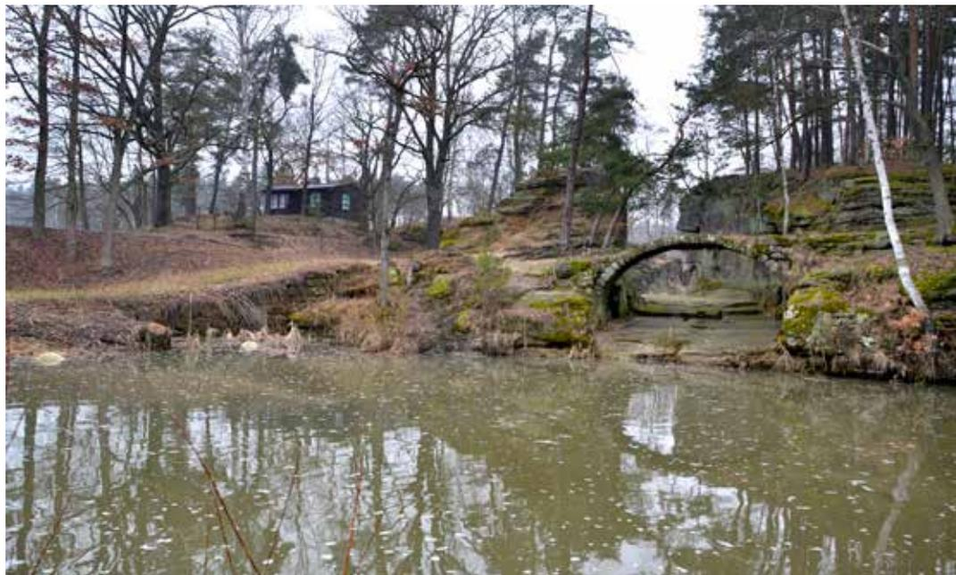
Fig. 4.90: Stvolínky, Mlýnský/Hrázský Pond – the main outlet of the pond with a bridge; to the left of it, a safety spillway. Photograph by Miroslav Kolka, 2013.
