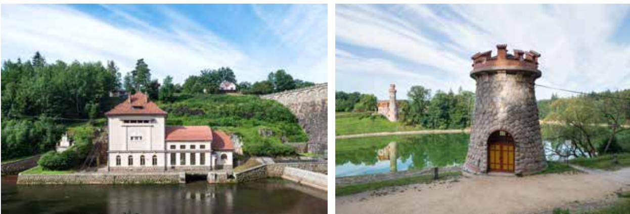
*Fig. 4.63: The Les Království dam (1910–1919) – on the left, the hydroelectric power plant building. On the right, the valve tower to control bottom outlets in the left by-pass tunnel; in the background, the dam keeper's house. Photograph by Viktor Mácha, 2020.*
