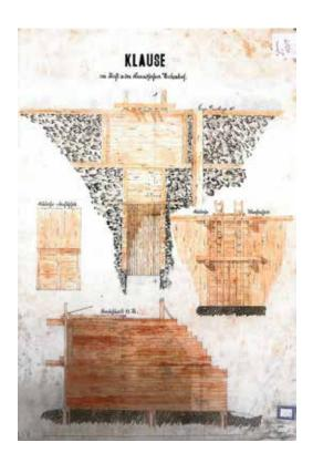
Fig. 5.308: Rudolf Rieger's diagram from 1863 with the original splash dam on Splavský Brook (taken from: SZA, Olomouc branch, inv. No. 1059.
