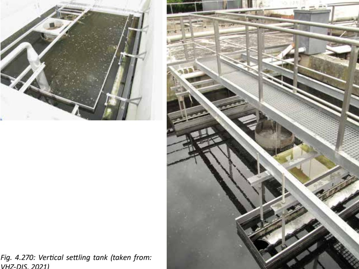
Fig. 4.270: Vertical settling tank (taken from: VHZ-DIS, 2021)
