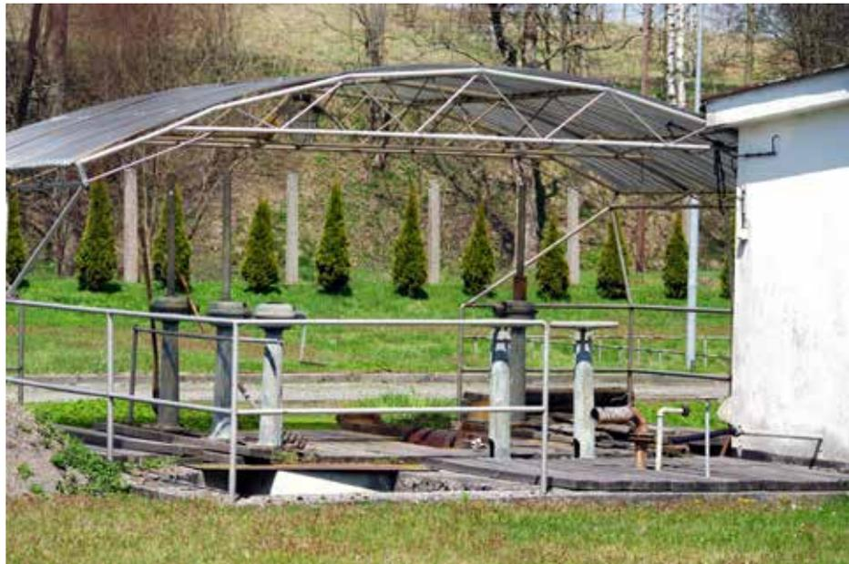
*Fig. 4.262: Coarse screen and inflow into the wastewater treatment plant with the control of gate valves. Photograph by Miloš Rozkošný, 2021.*
