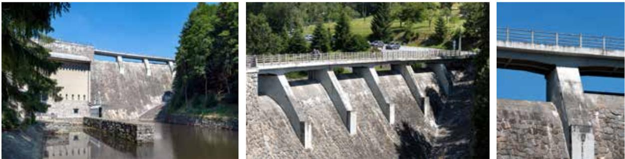
Fig. 4.50: The Pastviny dam (1933–1938) – masonry gravity dam. The last masonry-built dam in the Czech Republic to this day. In the pictures, there is an uncontrolled crown spillway with six bays having different overflow edge levels. Water is diverted through a chute into a stilling basin which is shut by a stepped sill. Photograph by Viktor Mácha, 2020.
