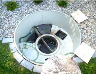
Fig. 4.281: Examples of domestic wastewater treatment plants (on the left, taken from: the Ekočov, s.r.o. archive, on the right, Rozkošný, 2012).
