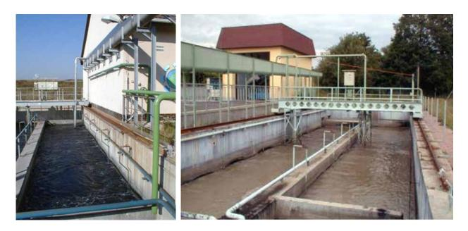
Fig. 4.265: Horizontal chamber sand trap (taken from: the TGM WRI archive).
