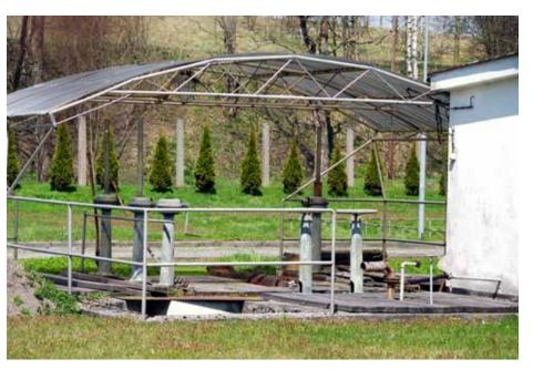
Fig. 4.262: Coarse screen and inflow into the wastewater treatment plant with the control of gate valves. Photograph by Miloš Rozkošný, 2021.
