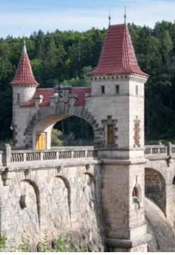
Fig. 4.62: The Les Království dam (1910–1919) – masonry gravity dam. Photograph by Viktor Mácha, 2020.
