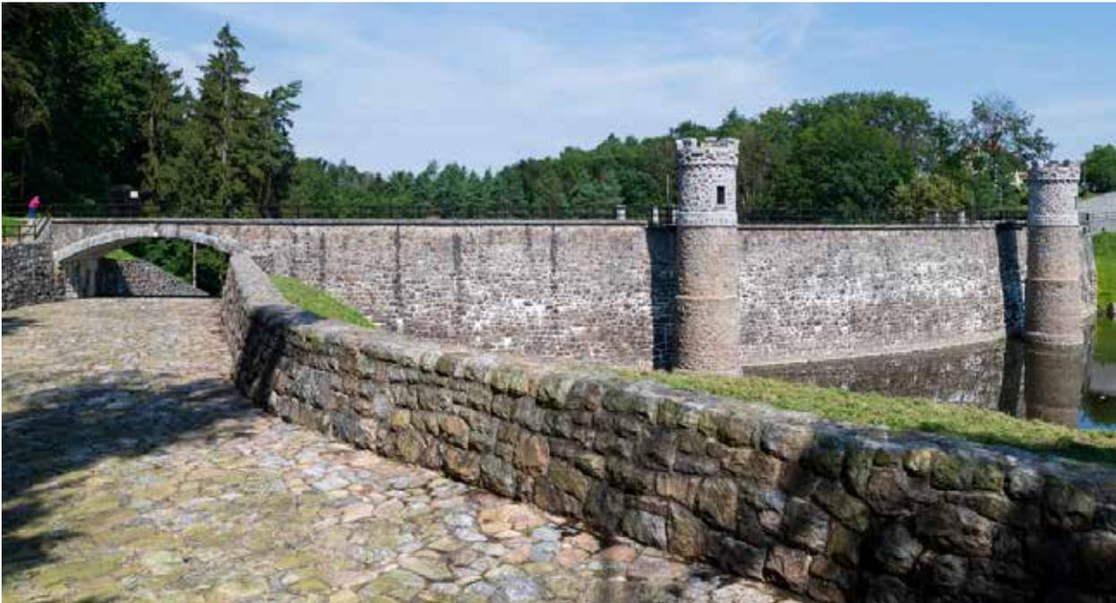
*Fig. 4.35: The Pařížov dam (1909–1913) – overflow edge of the side safety spillway and drop structure which behind the bridge follows the cascade. Photograph by Viktor Mácha, 2020.*
