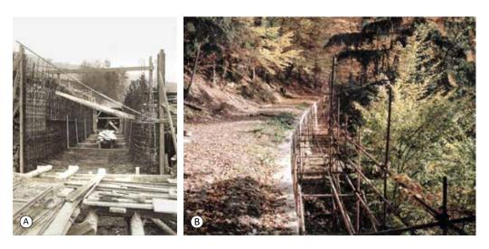
Fig. 4.173: Spálov SHPP – reinforced concrete supply channel: (A) reinforcement procedure in 1925. Taken from: VČE, 2000; (B) view from the channel ceiling in 1998 during reconstruction. On the right, photograph by Brno University of Technology, Faculty of Civil Engineering, 1998.
