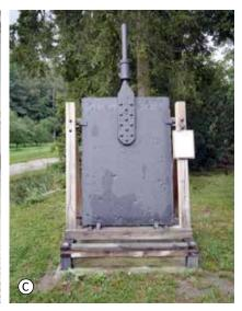
Fig. 4.49: The Jevišovice dam (1884–1896) – masonry gravity dam. (A) bottom outlets of the dam which constitute three tunnels; (B) control of operational valves of bottom outlets located at the crest of the dam which was originally outdoor, only later there was a structure built above it; (C) one of the original outlet valves, nowadays located under the dam. Photograph by Michaela Ryšková, 2020.
