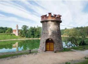
Fig. 4.63: The Les Království dam (1910–1919) – on the left, the hydroelectric power plant building. On the right, the valve tower to control bottom outlets in the left by-pass tunnel; in the background, the dam keeper's house. Photograph by Viktor Mácha, 2020.
