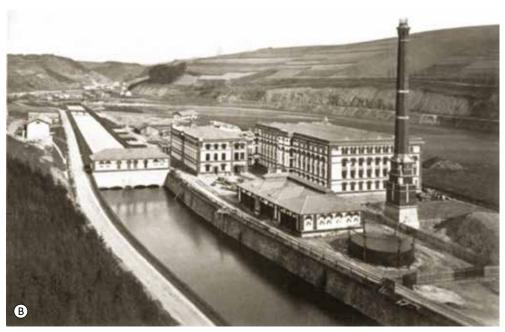
Fig. 4.158: Železný Brod – current situation of the derivation channel-type small hydroelectric power plant: (A) current layout after the demolition of the original machine room and subsequent complete reconstruction with a new machine room at the end of the derivation channel. The diagram was created on the basis of the ČÚZK data, 2021; (B) historic layout with the original location of the machine room from 1897. Photo archive of the company Vodní elektrárna Železný Brod, a.s.
