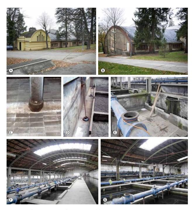
Fig. 5.318: Plzeň – the Puech-Chabal filtration building: (A) main entrance and the highest situated north-eastern hall; (B) the lowest situated south-western hall; (C) and (D) documentation from the course of cleaning of individual tanks; (E) - (G) overall views during current operation. Photograph by Jan Mikač, 2015, and Michaela Ryšková, 2020.
