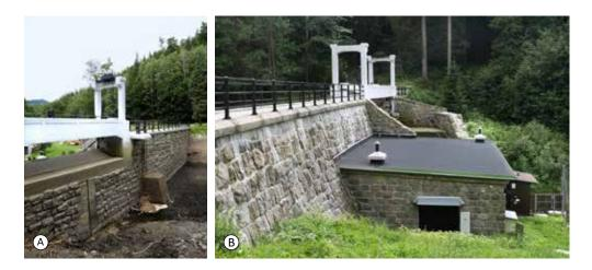
Fig. 4.156: Rudolfov II SHPP: (A) upstream slope of the dam with an inlet structure; (B) SHPP machine room. Photograph by Michaela Ryšková, 2021.
