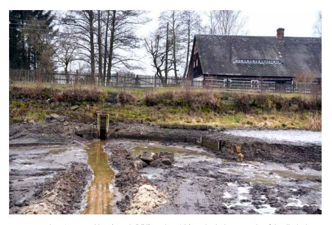
Fig. 4.88: Markvartice near Jablonné v Podještědí, Markvartický Pond – the bottom outlet of the idle discharge with a monk outlet, upstream face with typical revetment from sandstone blocks; state after the pond drawdown. Photograph by Miroslav Kolka, 2014.
