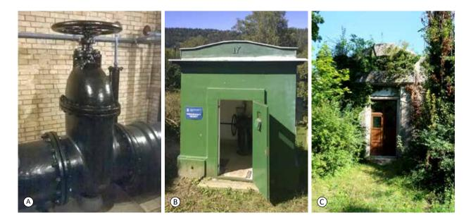
Fig. 3.3: 1st Březová aqueduct (A) aqueduct supply valve; (B) gate valve chamber; (C) entrance to the Holé Hory 2 water tank; cast iron long-distance aqueduct for drinking water (57 km), preserved in its original form with the exception of the addition of a remote control system to operate the machinery. Photograph (A,B) by Miriam Dzuráková, 2018 and (C) by David Honek, 2019.
