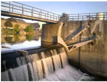
Fig. 4.133: Radial gate weir. Diagram by Radka Račoch and Michaela Mrvová, 2021 (modified according to Gabriel et al., 1989). On the right, a radial gate weir in Přerov. Photograph from the Brno University of Technology archive, 2019.
