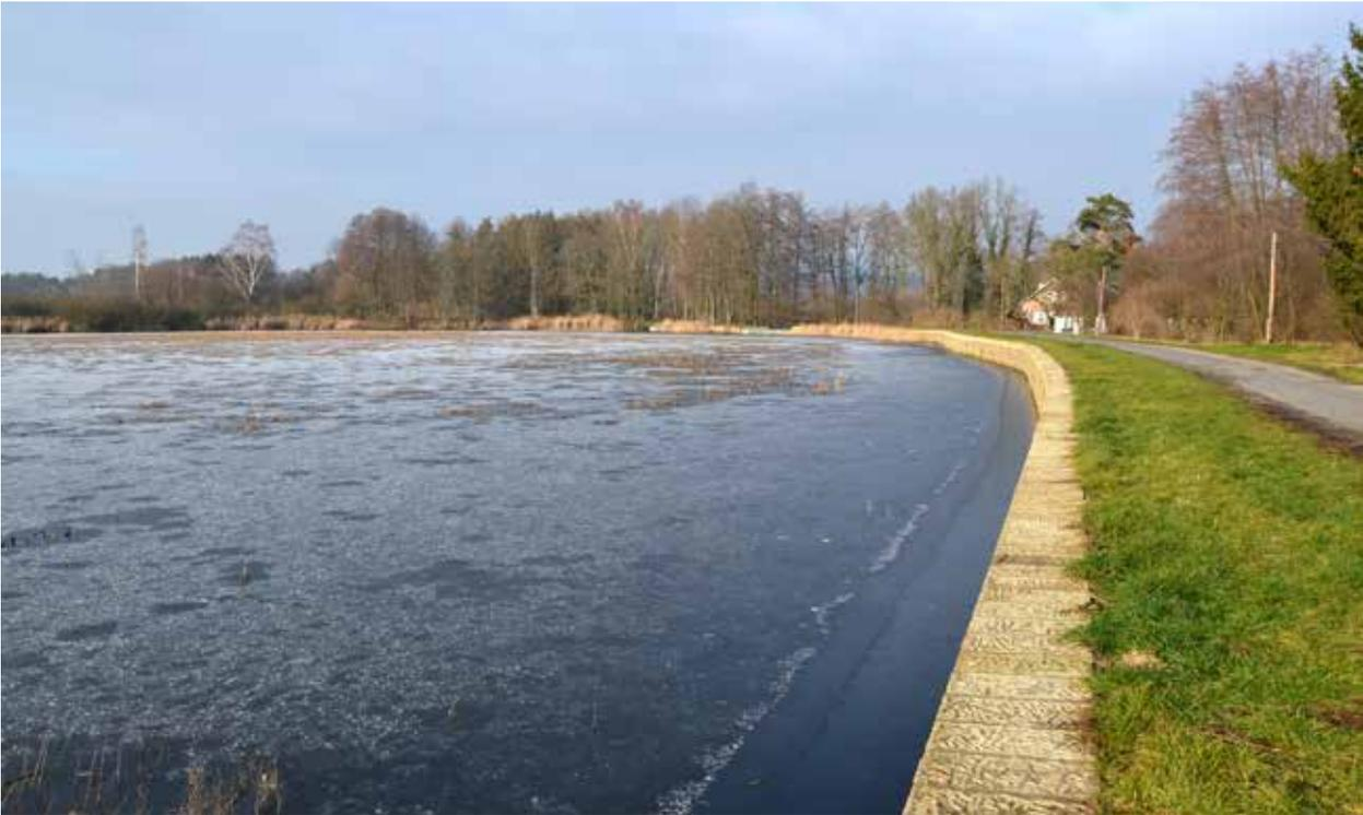
*Fig. 4.75: Holany, Holanský Pond – a concave shape of a dam with a restored upstream wall from sandstone blocks. Photograph by Miroslav Kolka, 2018.*
