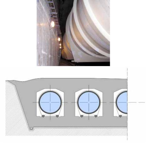
Fig. 4.177: Dalešice PSHPP – pressure turbine steel pipeline positioned in the gallery. Photograph by Brno University of Technology, Faculty of Civil Engineering, 2015. Diagram by Radek Míšanec, 2021 (modified according to: Hynková, 1984).
