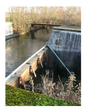
Fig. 4.117: Austria, Laa an der Thaya — an iron aqueduct on a race from the Dyje River. Photograph by Milena Forejtníková, 2019.
