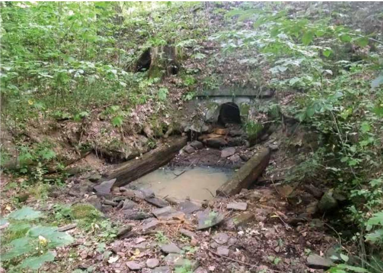
*Fig. 4.86: The original bottom outlet of the extinct Nový Pond near Zbýšov with preserved relics of a pipeline pit and stilling basin. Photograph by Jindřich Frajer, 2020.*
