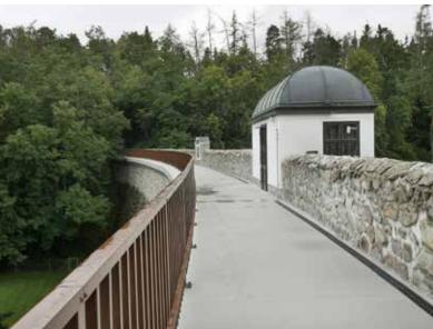
Fig. 5.323: The Jevišovice dam – structure for handling bottom outlets. Photograph by Michaela Ryšková, 2020.
