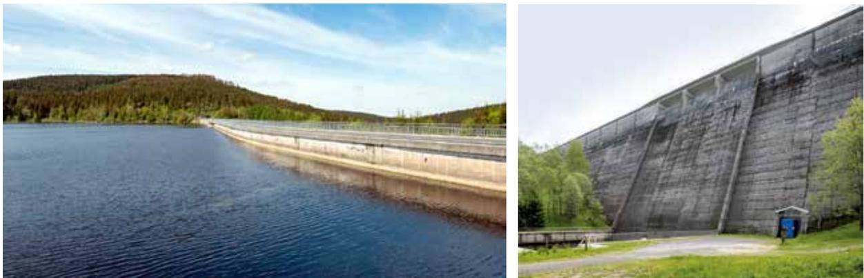
Fig. 4.43: The Fláje dam (1951–1963) – buttress dam. Photograph by Viktor Mácha, 2020.
