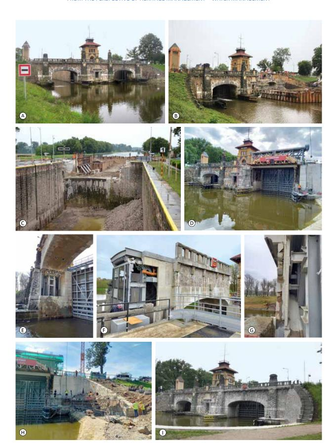
Fig. 5.302: Hořín – lock in the course of reconstruction: (A) state before the reconstruction; (B) and (C) dismantling of original structures and stone cladding; (D) to (F) new moveable bridge and lock chamber structures; (G) and (H) installation of the original facing on a new reinforced concrete structure. Photograph by Otakar Hrdlička, 2021; (I) current lock appearance. Photograph by Michaela Ryšková, 2021.
