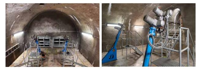
Fig. 4.34: The Pařížov dam (1909–1913) – handling of operational radial gates of bottom outlets (DN1200) located in the by-pass tunnel. Photograph by Viktor Mácha, 2020.
