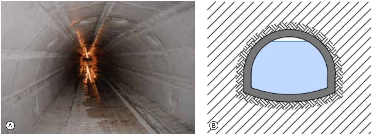
Fig. 4.174: Spálov SHPP – free-surface gallery: (A) view of the gallery after reconstruction with the use of geomembrane. Photograph taken from: VČE, 2000; (B) diagram by Radek Míšanec, 2021 (modified according to: ZČE, 2000).
