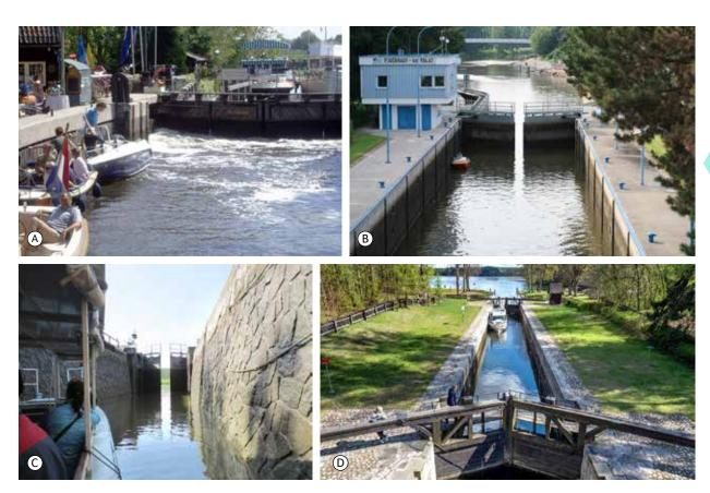
Fig. 4.103: Examples of lock chambers: (A) Netherlands, filling of a lock chamber by a gate by-pass; photograph by V. Forejtník, 2007; (B) Poděbrady, a lock chamber with steel gates filling by-pass channels openings; photograph by Miriam Dzuráková, 2021; (C) a lock on the Baťa Canal on the lower water, Cyclopean masonry; the TGM WRI archive, 2012; (D) — Poland, a lock with wooden gates on the Augustów Canal; photograph from Milena Forejtníková's personal archive.
