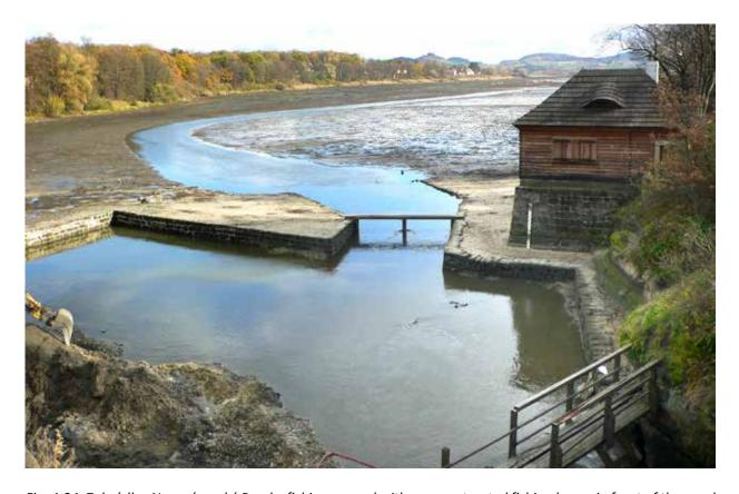
Fig. 4.94: Zahrádky, Novozámecký Pond – fishing ground with a reconstructed fishing house in front of the pond sluice gate outlet, walled by sandstone blocks. Photograph by Miroslav Kolka, 2006.
