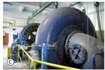
Fig. 4.207: Weisshuhn race and the paper mill hydroelectric power plant: (A) upper race trough with a railwayman's house; (B) aqueduct at the crossing with Kamenný Brook; (C) the interior of a hydroelectric power plant machine room with a Francis turbine and a generator. Photograph by Radka Račoch, 2021 (A) and (B), Miriam Dzuráková, 2019 (C).
