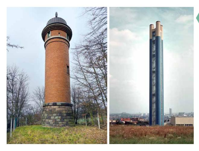
Fig. 4.249: Relief and stand-pipe towers of aqueducts: (A) Letovice – relief tower of the 1st Březová conduit to supply drinking water to Brno. Photograph by Michaela Ryšková, 2016; (B) Prague – stand-pipe tower Děvín built according to architect Karel Hubáček's design, SIAL. Photograph from the PVK archive, f. Fotoarchiv PVK, kt. N 8, sign. B 951b.
