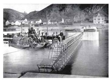
Fig. 4.129: On the left, a needle weir. Diagram by Radka Račoch and Radek Bachan, 2021 (modified according to: Kratochvíl, 1947). On the right, a needle weir in Klecany (taken from: Klír, 1908.)
