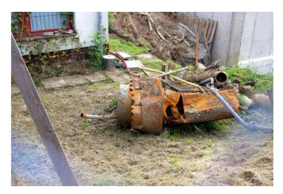
Fig. 5.326: The fitting of the secondary settling tank damaged during the renovation of the water treatment plant. Photograph by Miloš Rozkošný, 2021.
