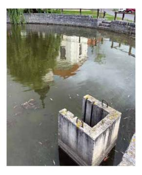
Fig. 4.85: Ostrov u Stříbra – village square SWR with concrete open double monk outlet. Photograph by Renata Pavelková, 2021.
