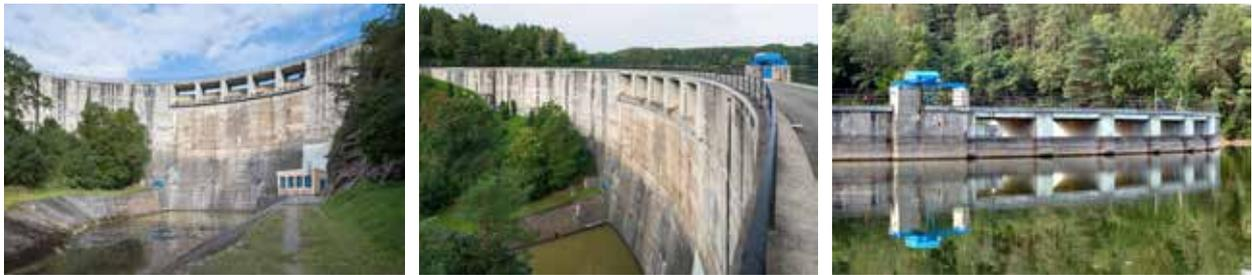
Fig. 4.45: The Vrchlice dam (1966–1970) – arch dam. Photograph by Viktor Mácha, 2020.
