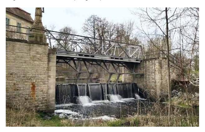
Fig. 4.131: A shutter weir with overhead bridge in Křimice. Photograph from the Brno University of Technology archive, 2018.
