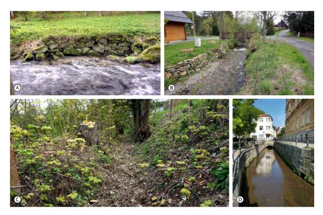
Fig. 4.115: Building material – stone – Jeseníky (Karlov, Malá Morávka): (A) assembled stone, durability verified over time; (B) newer variant of assembled stone; (C) stone race which is no longer there; Chrudim: (D) stone walls of a water canal in an intravilan. Photograph by David Honek, 2020.
