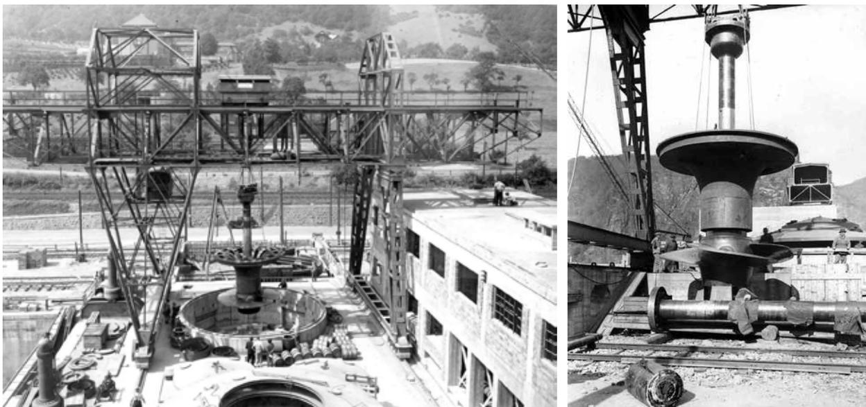
Fig. 4.200: Střekov HPP – a machine set with a vertical Kaplan turbine – installation of a runner (taken from: the Povodí Labe, s.p. [Elbe River Basin] archive).
