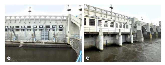
Fig. 4.165: Kolín SHPP: (A) inlet structure; (B) outlet structure. Photograph by Brno University of Technology, Faculty of Civil Engineering, 2015.
