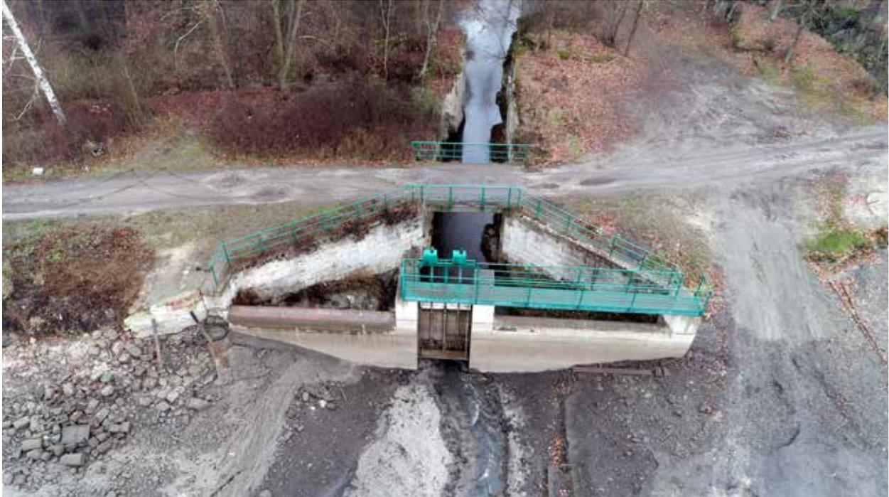
*Fig. 4.80: Holany, Holanský Pond – the main outlet with a discharge to the sandstone rock gully. Photograph by J. Vidman, 2018.*
