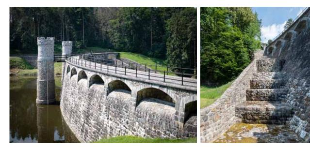
Fig. 4.36: The Pařížov dam (1909–1913) – On the left, the view on the crown safety spillway from the upstream side. On the right, the view from the downstream side on the crown spillway cascade. Photograph by Viktor Mácha, 2020.
