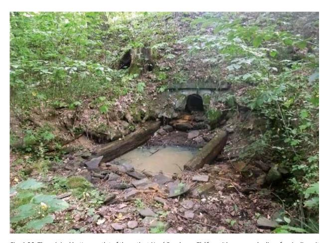
Fig. 4.86: The original bottom outlet of the extinct Nový Pond near Zbýšov with preserved relics of a pipeline pit and stilling basin. Photograph by Jindřích Frajer, 2020.
