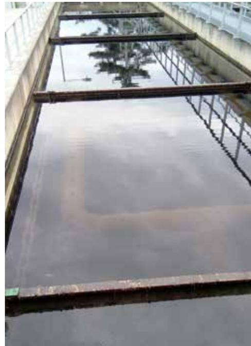
*Fig. 4.267: Horizontal settling tank. Photograph by Miloš Rozkošný, 2021.*
