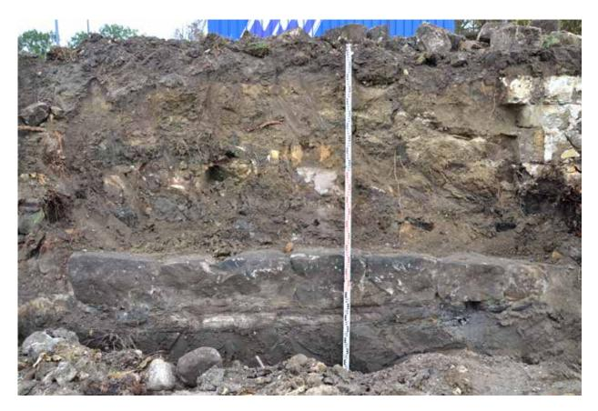
Fig. 4.78: Holany, Holanský Pond – construction of the dam with the revetment of the upstream face, the sandstone masonry is founded on the beam grid from the beginning of the 16th century. Photograph by Miroslav Kolka, 2018.
