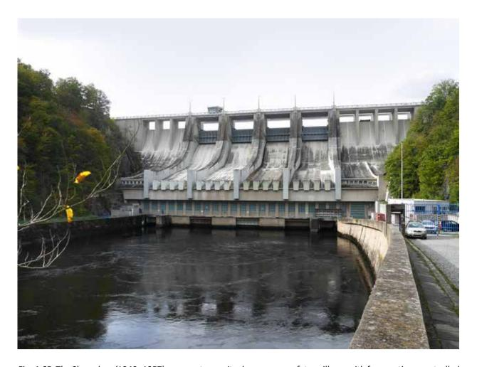
Fig. 4.65: The Slapy dam (1949–1957) – concrete gravity dam, crown safety spillway with four sections controlled by a lifting gate. Photograph by Viktor Mácha, 2021.
