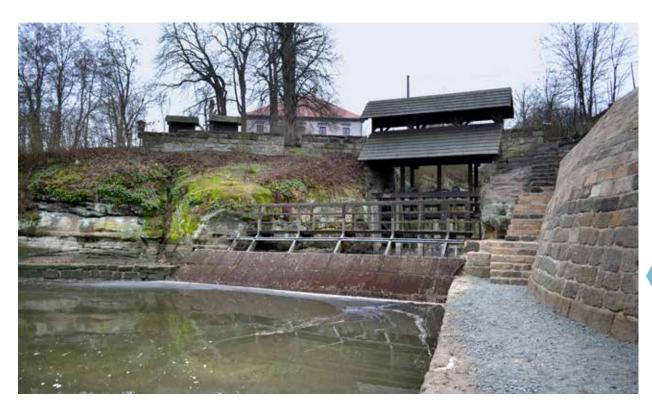
Fig. 4.87: Zahrádky, Novozámecký Pond – outlet with an open tailrace and massive sluice gate beam structure with a foot bridge, roof and racks; all structures are installed into grooves in sandstone walls. Photograph by Miroslav Kolka, 2015.
