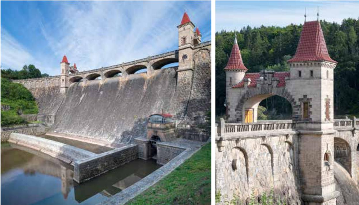
*Fig. 4.62: The Les Království dam (1910–1919) – masonry gravity dam. Photograph by Viktor Mácha, 2020.*
