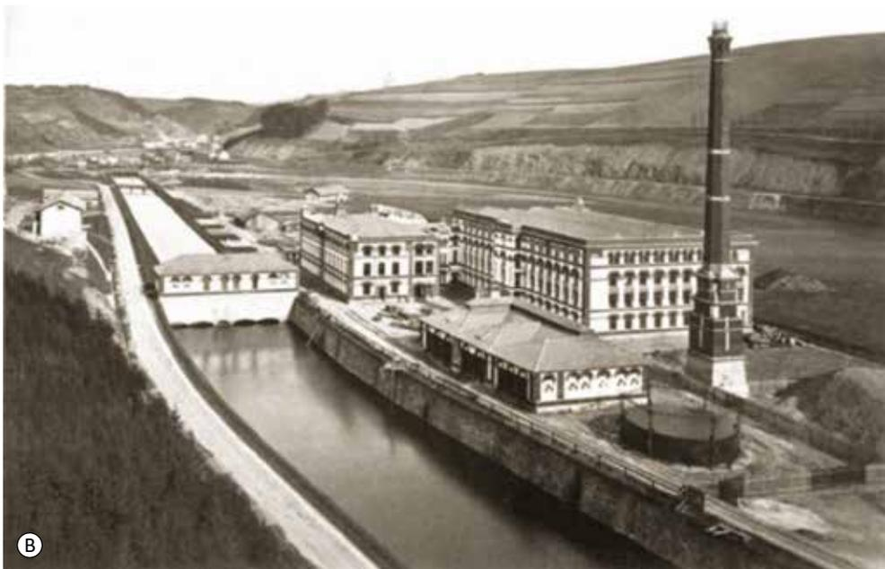
Fig. 4.158: Železný Brod – current situation of the derivation channel-type small hydroelectric power plant: (A) current layout after the demolition of the original machine room and subsequent complete reconstruction with a new machine room at the end of the derivation channel. The diagram was created on the basis of the ČÚZK data, 2021; (B) historic layout with the original location of the machine room from 1897. Photo archive of the company Vodní elektrárna Železný Brod, a.s.
