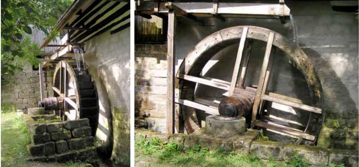
Fig. 4.189: Overshot bucket water wheel. Photograph by Radim Urbánek, 2006.
