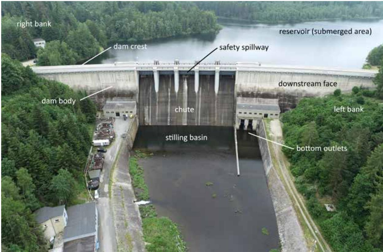
Fig. 4.25: Definitions of basic terms – the Kružberk dam (1948–1955). Photograph by Radek Bachan, 2021.
