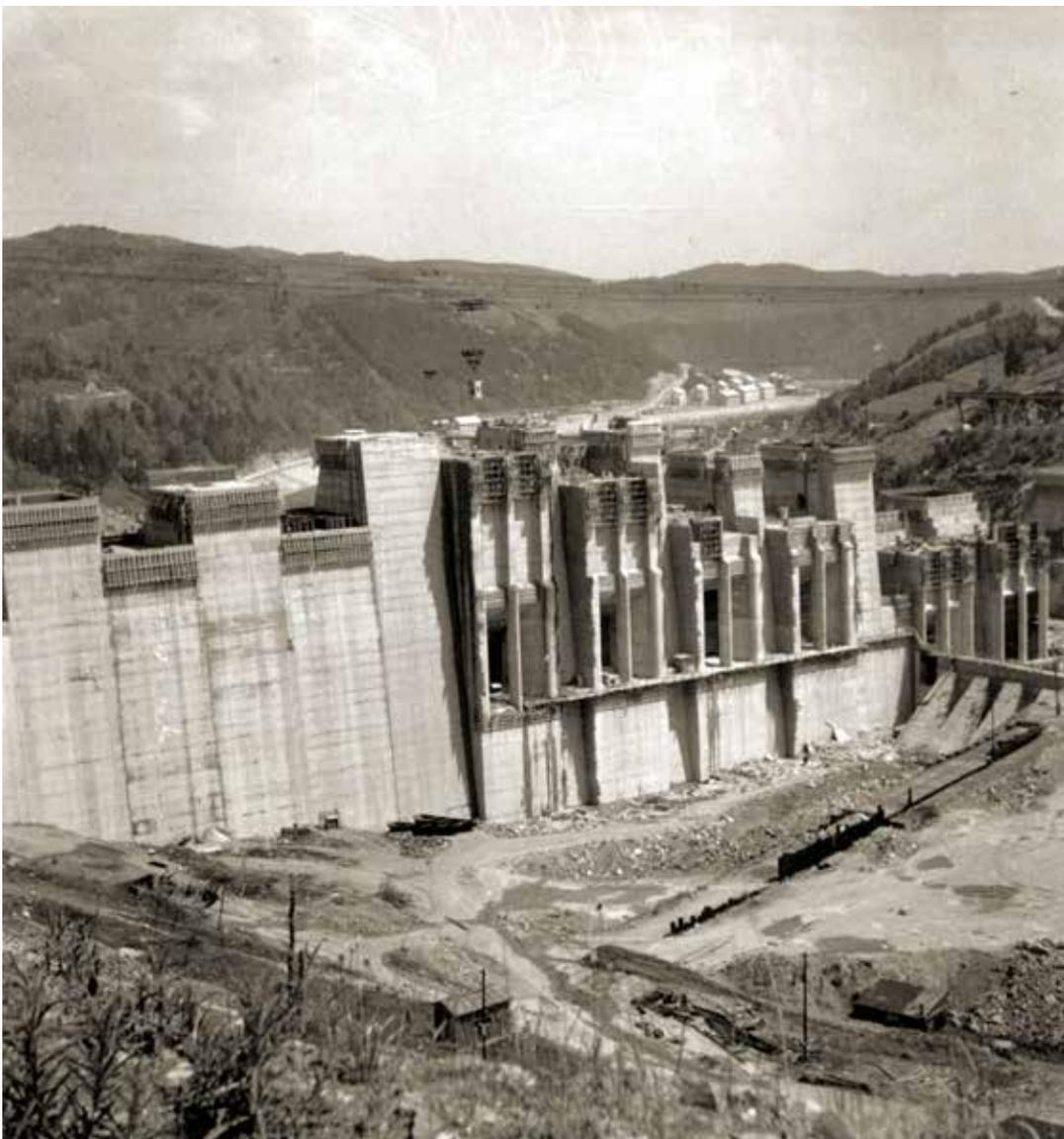
*Fig. 4.168: Orlik HS – under construction, detail of blocks with inlets to the HPP. Photograph by Brno University of Technology, Faculty of Civil Engineering.*
