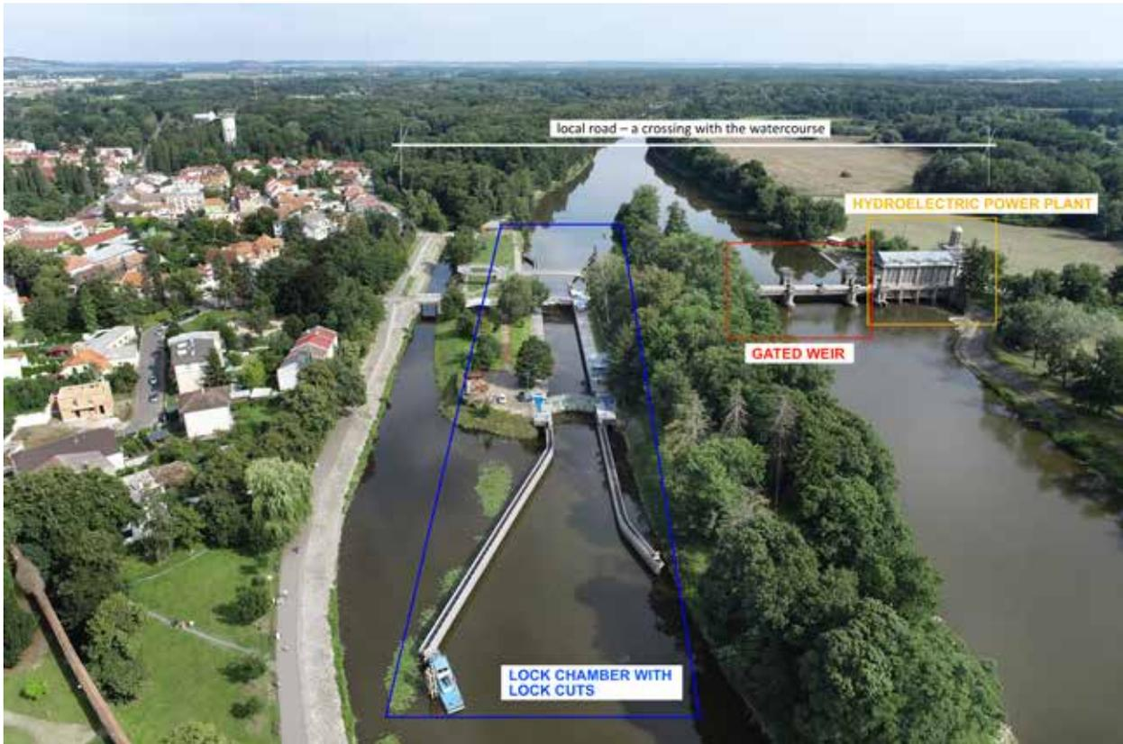
*Fig. 4.144: The Poděbrady navigation lock – functional complex elements. Photo by Radek Bachan, 2021.*
