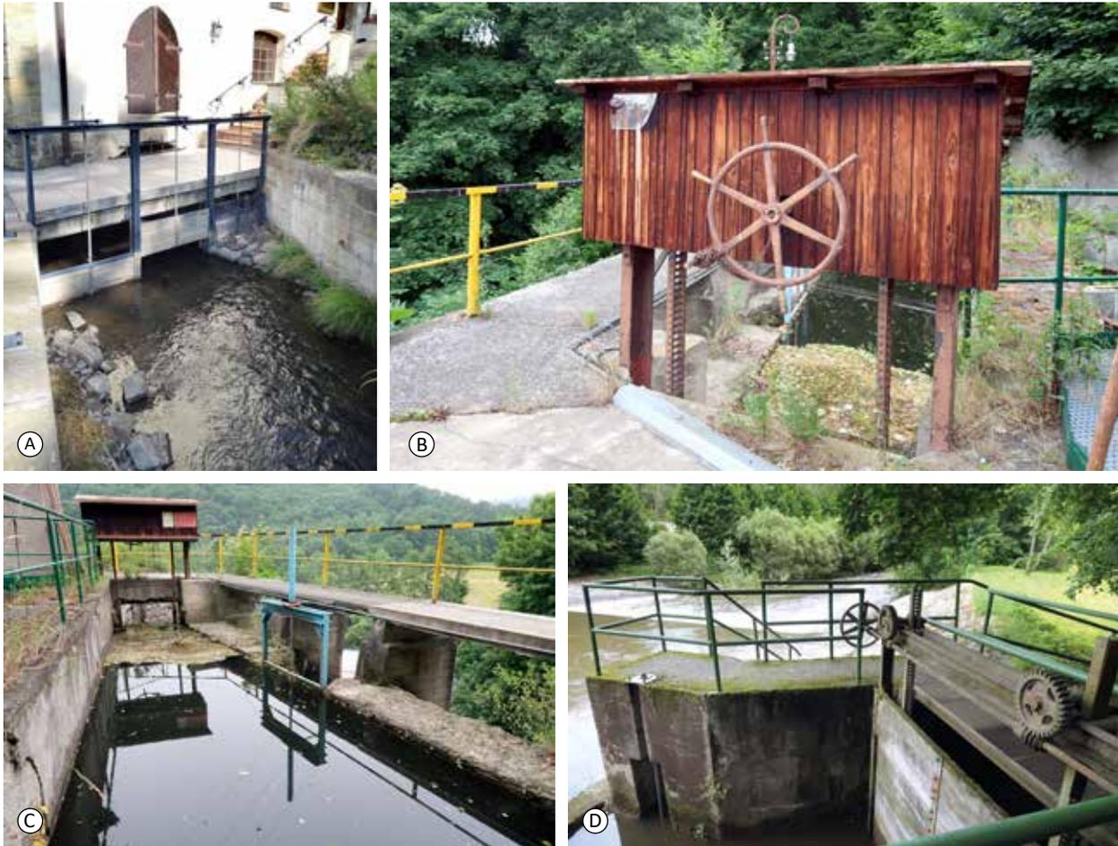
*Fig. 4.118: Control structures details: (A) Chrudim – wood, hand-operated sluice gates; (B) the Weisshuhn Canal, an originally hand-operated sluice gate converted into electrically-powered; (C) the same place, right-bank residual outflow operated hydraulically; (D) mechanism for manual control of sluice gates from the side. Photograph by Radka Račoch, 2021.*
