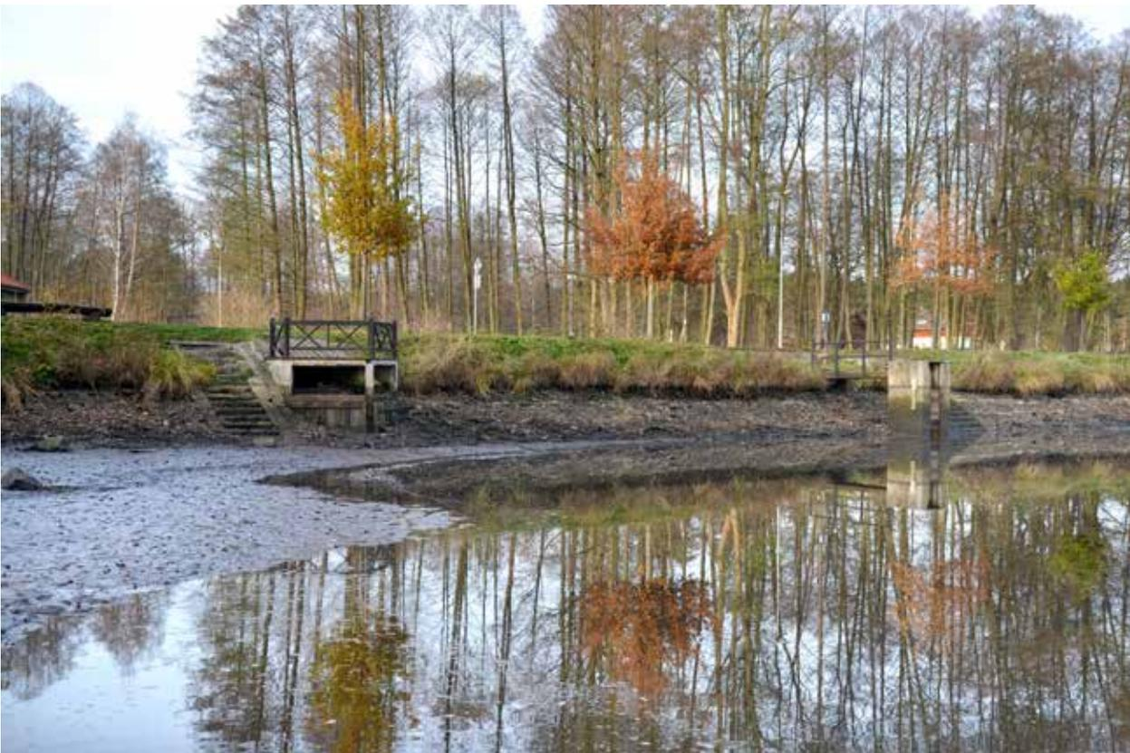
*Fig. 4.76: Hradčany, Hradčanský Pond – a straight dam with a main outlet (on the right) and a discharge to the race to the extinct mill (on the left); state after the pond drawdown. Photograph by Miroslav Kolka, 2017.*
