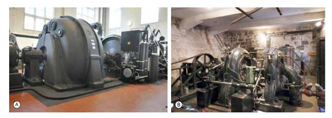
Fig. 5.305: Rudolfov SHPP – machine room interior: (A) Rudolfov I SHPP with the Pelton turbine; (B) Rudolfov II SHPP with the Francis turbine. Photograph by Petr Freiwillig, 2014 (A), 2013 (B).
