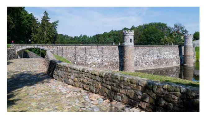
Fig. 4.35: The Pařížov dam (1909–1913) – overflow edge of the side safety spillway and drop structure which behind the bridge follows the cascade. Photograph by Viktor Mácha, 2020.
