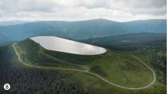
Fig. 3.21: Dlouhé stráně PSHPP: (A) lower reservoir; (B) upper reservoir; an example of upper and lower reservoirs with controversial landscape/urbanistic value and a substantial impact on the appearance of the location. The upper reservoir has had a major impact on the panorama of the High Jeseníky mountains due to the removal of the hill's original summit, which has been levelled. Photograph by (A) David Honek, 2019, (B) by Shutterstock, 2021.
