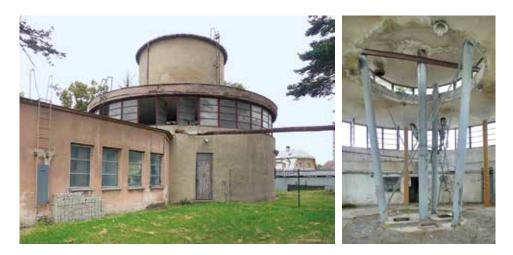
Fig. 4.247: Krnov — elevated water tank on the premises of the Karnola plant. An elevated water tank with unknown date of origin and authorship intended for non-potable water for the Karnola textile plant. A low-height water structure with a cylindrical tank carried by steel shanks and an architecturally designed casing, composed of two cylinders of different scales and broken by two horizontal ribbon windows. It was demolished in 2020. Photograph by Michaela Ryšková, 2013.
