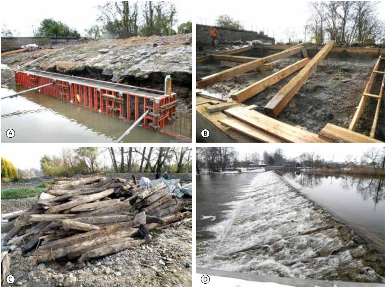
Fig. 5.303: Znojmo-Oblekovice – reconstruction of the weir in Oblekovice on the Dyje River: (A) Foundation of a new weir heel, October 2018; (B) Replacement of the weir body beam grid, November 2018; (C) original parts of the wooden beam structure; (D) reconstruction completed, January 2019. Photograph by Miriam Dzuráková, 2018-2019.
