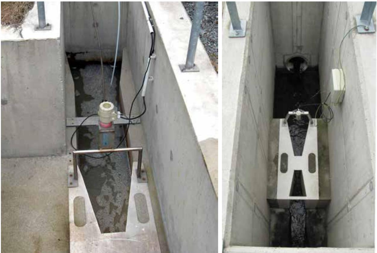
Fig. 4.279: The Purshall flume, an ultrasound sensor for the measurement of water flow (taken from: the TGM WRI archive).
