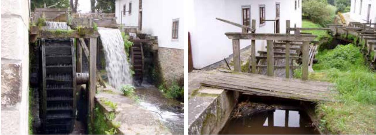
Fig. 4.113: Ratibořice, wooden elements of the mill race at Granny's valley. Photograph by Milena Forejtníková, 2010.
