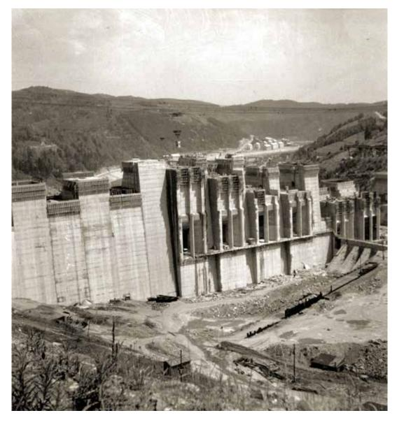
Fig. 4.168: Orlík HS – under construction, detail of blocks with inlets to the HPP. Photograph by Brno University of Technology, Faculty of Civil Engineering.
