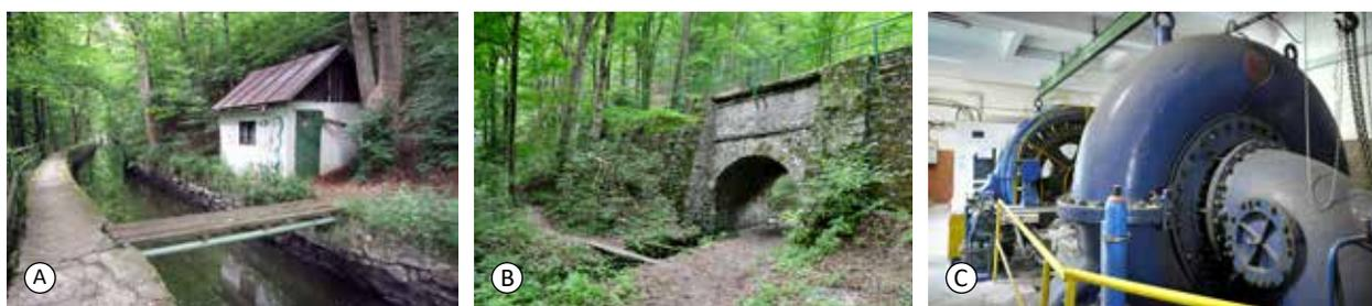
Fig. 4.207: Weisshuhn race and the paper mill hydroelectric power plant: (A) upper race trough with a railwayman's house; (B) aqueduct at the crossing with Kamenný Brook; (C) the interior of a hydroelectric power plant machine room with a Francis turbine and a generator. Photograph by Radka Račoch, 2021 (A) and (B), Miriam Dzuráková, 2019 (C).
