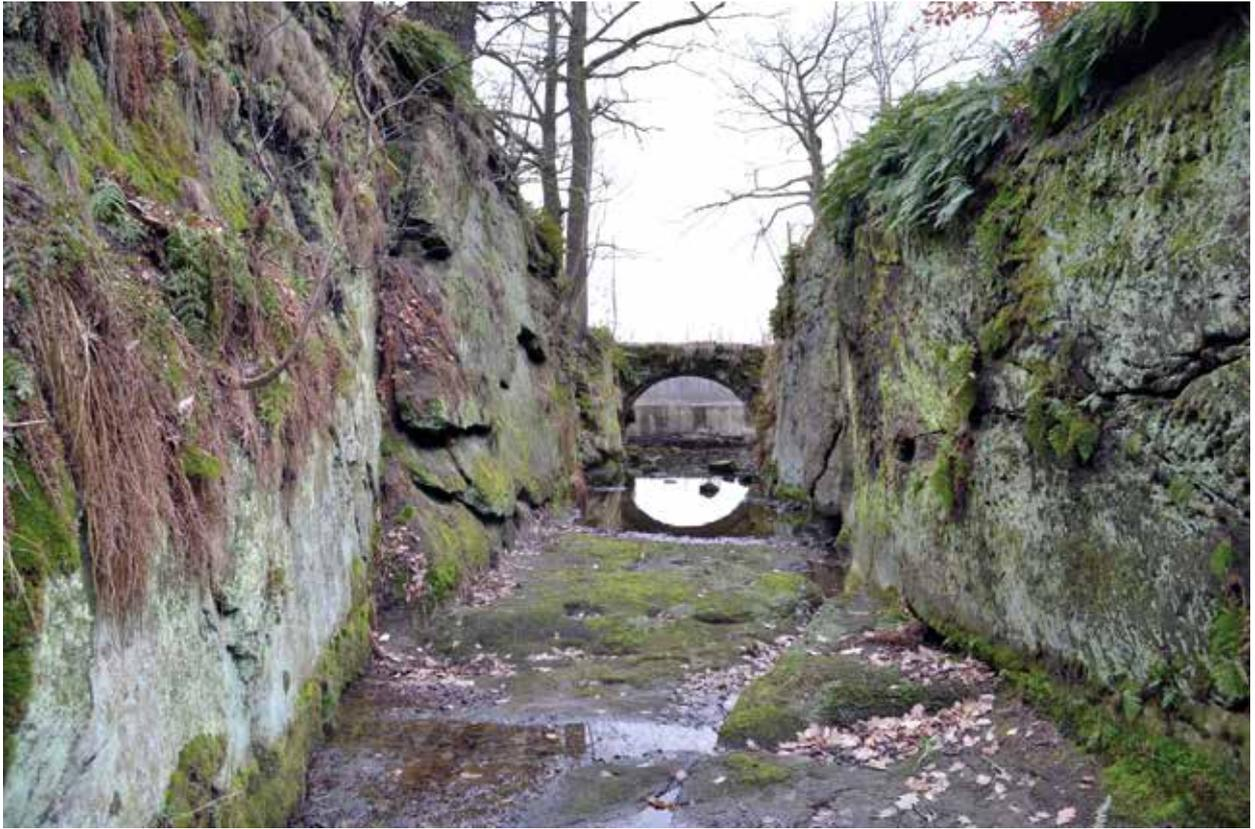
*Fig. 4.91: Stvolínky, Dolanský Pond – a rock gully of the safety spillway; in the background a bridge in the dam route. Photograph by Miroslav Kolka, 2016.*
