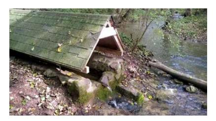
Fig. 4.231: Ochoz u Brna – spring tank (Kaprálova studánka) catching underground water springs in close proximity to the Říčka River. Photograph by David Honek, 2014.
