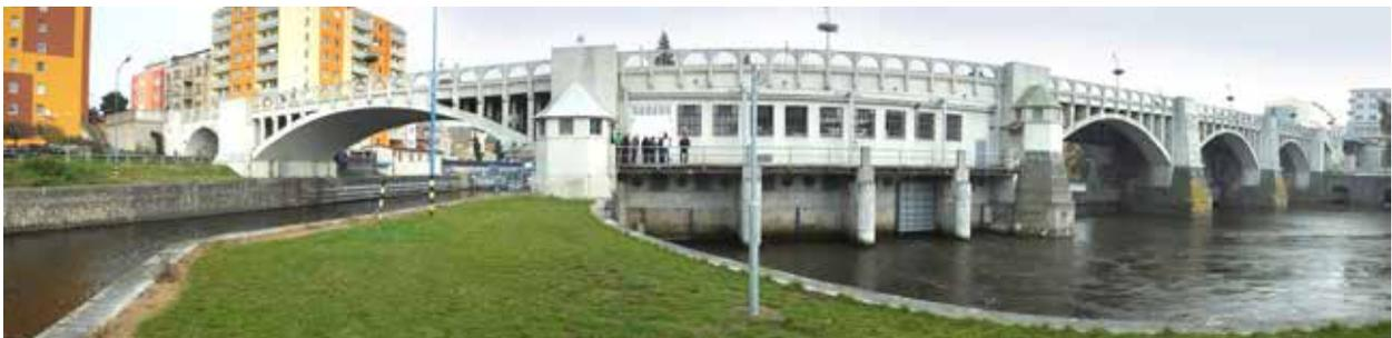
Fig. 4.155: Kolín SHPP – a view from the area downstream of the weir of the machine room and the outlet part of the small hydroelectric power plant (on the left) and three sections of the roller drum weir (on the right). Photograph by Brno University of Technology, Faculty of Civil Engineering, 2014.
