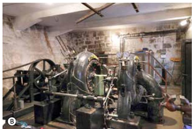
Fig. 5.305: Rudolfov SHPP – machine room interior: (A) Rudolfov I SHPP with the Pelton turbine; (B) Rudolfov II SHPP with the Francis turbine. Photograph by Petr Freiwiligg, 2014 (A), 2013 (B).
