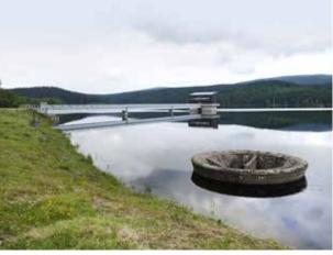
Fig. 4.54: The Josefův Důl dam (1976–1982) – earthfill dam, shaft safety spillway. Photograph by Michaela Ryšková, 2020.
