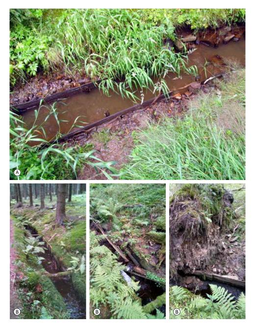
Fig. 5.310: Blatná Water Ditch – damaged sections of the water ditch: (A) affected by erosion and washing out; (B) endangered and damaged by woody plants in the proximity of the race trough. Photograph by Miloš Rozkošný, 2020.
