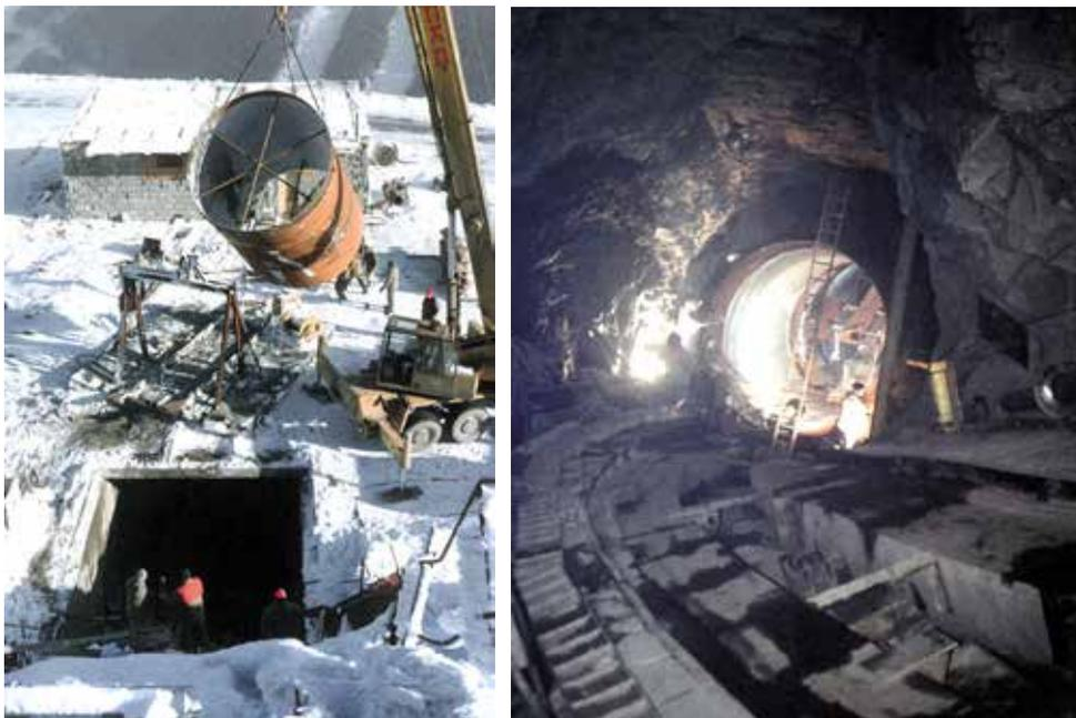
Fig. 4.175: Dlouhé stráně PSHPP – positioning of steel armour into the inlet gallery of turbines (taken from: Höll, 1997).
