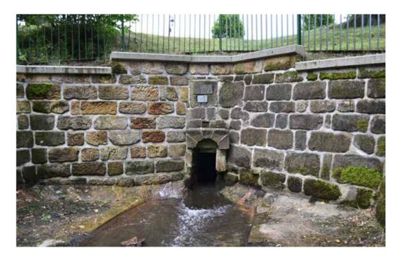
Fig. 4.89: Hamr na Jezeře, Hamerský Pond – downstream face of the dam with the bottom outlet, dated 1821; state after the modern modifications of walls. Photograph by Miroslav Kolka, 2017.
