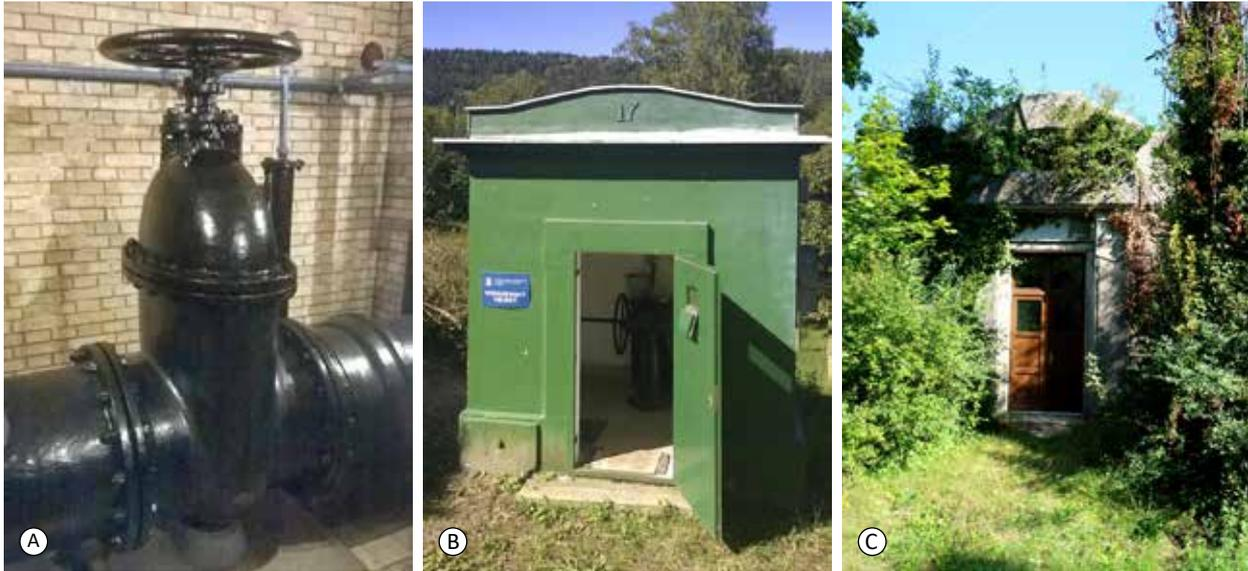
*Fig. 3.3: 1st Březová aqueduct (A) aqueduct supply valve; (B) gate valve chamber; (C) entrance to the Holé Hory 2 water tank; cast iron long-distance aqueduct for drinking water (57 km), preserved in its original form with the exception of the addition of a remote control system to operate the machinery. Photograph (A,B) by Miriam Dzuráková, 2018 and (C) by David Honek, 2019.*
