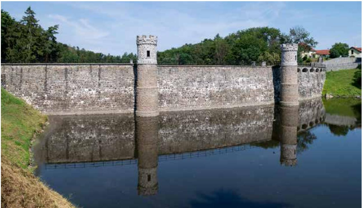
*Fig. 4.33: The Pařížov dam (1909–1913) – control towers on the upstream side of the dam for the handling of inspection slide gate valves. Photograph by Viktor Mácha, 2020.*
