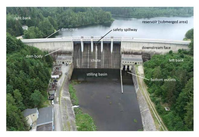
Fig. 4.25: Definitions of basic terms – the Kružberk dam (1948–1955). Photograph by Radek Bachan, 2021.
