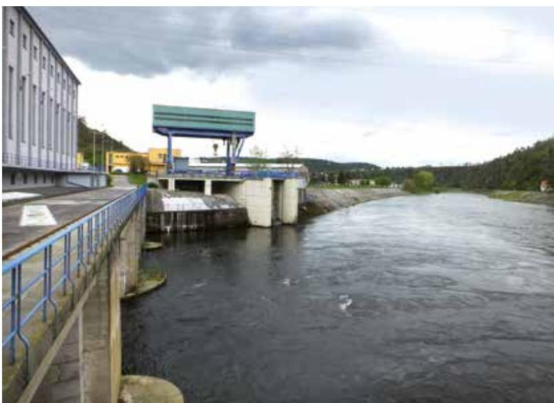
Fig. 4.186: Štěchovice PSHP with a shaft-type machine room. Photograph by Brno University of Technology, Faculty of Civil Engineering, 2019.
