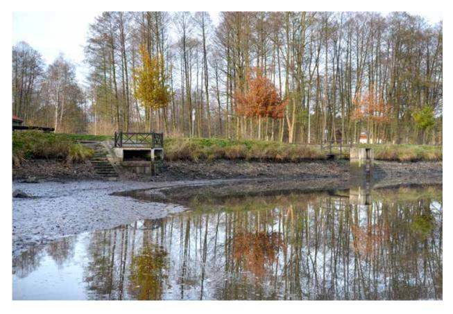
Fig. 4.76: Hradčany, Hradčanský Pond – a straight dam with a main outlet (on the right) and a discharge to the race to the extinct mill (on the left); state after the pond drawdown. Photograph by Miroslav Kolka, 2017.
