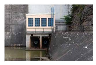
Fig. 4.48: The Vrchlice dam (1966–1970) – arch dam. On the left, operational Howell Bunger valve of bottom outlets. On the right, control equipment of Howell Bunger valves. Photograph by Viktor Mácha, 2020.
