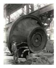
Fig. 4.202: Production of the Francis turbine runner for the Miřejovice SHPP (taken from: ČKD Blansko company materials).
