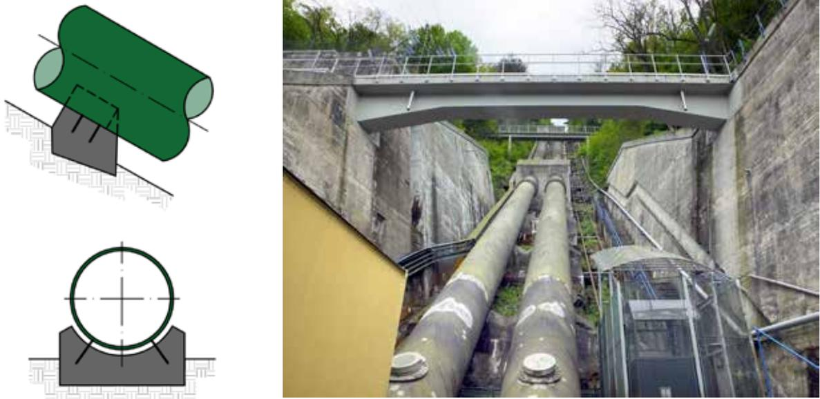
Fig. 4.178: Support block construction: (A) Diagram by Radka Račoch and Radek Bachan, 2021 (modified according to: Broža et al., 1990); (B) Štěchovice PSHPP – pressure pipeline with support and anchor blocks. Photograph by Brno University of Technology, Faculty of Civil Engineering, 2019.
