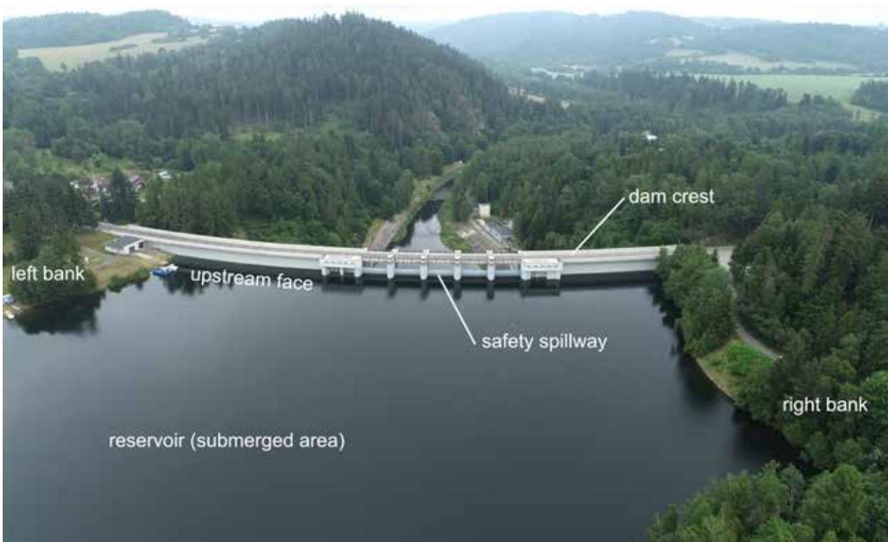
Fig. 4.26: Definitions of basic terms – the Kružberk dam (1948–1955). Photograph by Radek Bachan, 2021.
