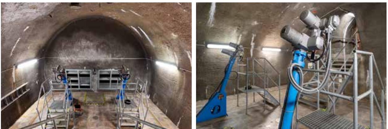
*Fig. 4.34: The Pařížov dam (1909–1913) – handling of operational radial gates of bottom outlets (DN1200) located in the by-pass tunnel. Photograph by Viktor Mácha, 2020.*
