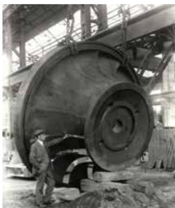
*Fig. 4.202: Production of the Francis turbine runner for the Miřejovice SHPP (taken from: ČKD Blansko company materials).*
