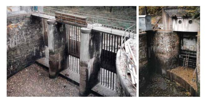
Fig. 4.167: Spálov derivation SHPP – inlet structure, state without water at the time of repair in 1998. Photograph by Brno University of Technology, Faculty of Civil Engineering, 1998.
