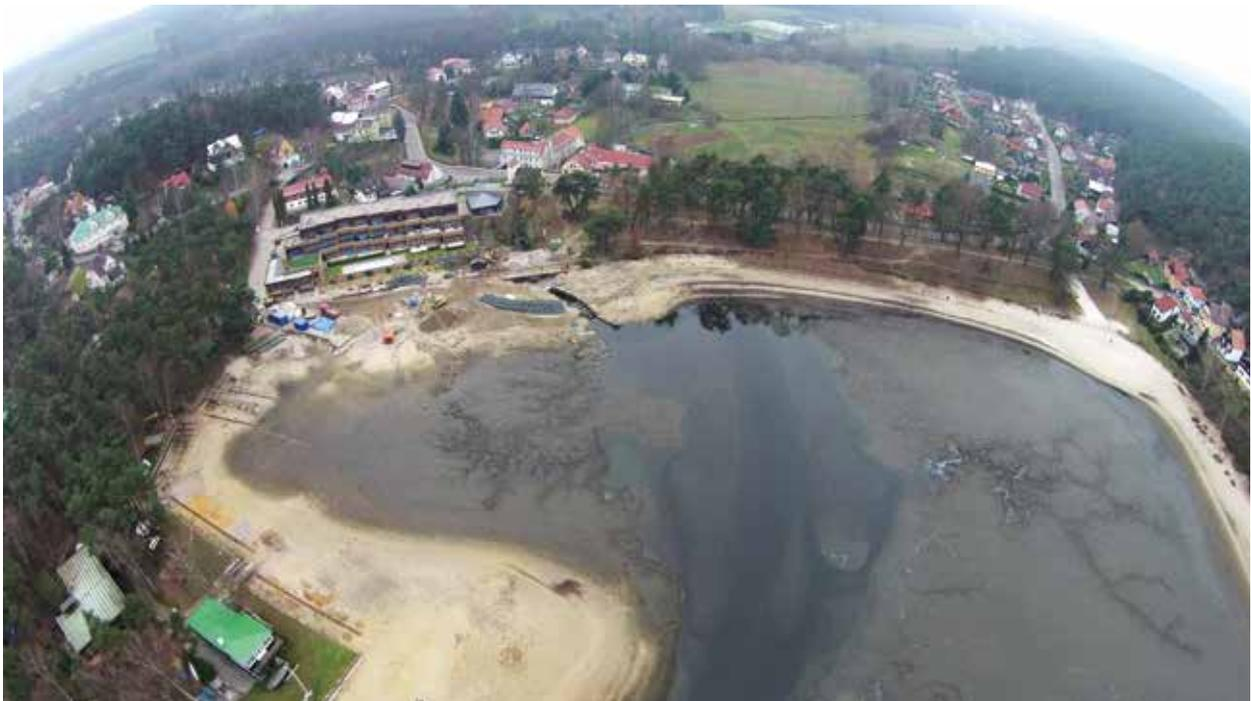
Fig. 4.74: Doksy – Staré Splavy, Máchův náhon – In the left part of the picture, a straight dam of a pond which consists of an outcrop of a sandstone bedrock with a basalt vein, in the middle part there is an outlet gully; state during the reconstruction of the outlet structure and the pond drawdown. Photograph by A. Kopecký, 2014.
