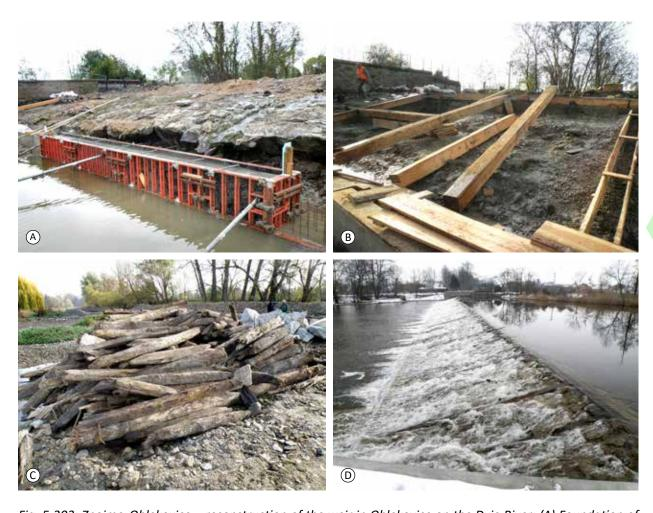
Fig. 5.303: Znojmo-Oblekovice – reconstruction of the weir in Oblekovice on the Dyje River: (A) Foundation of a new weir heel, October 2018; (B) Replacement of the weir body beam grid, November 2018; (C) original parts of the wooden beam structure; (D) reconstruction completed, January 2019. Photograph by Miriam Dzuráková, 2018-2019.
