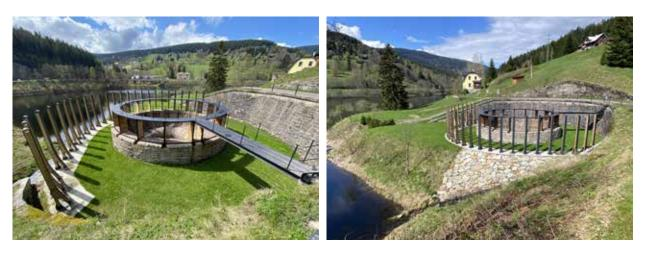
Fig. 4.53: The Labská dam (1910–1916) – masonry gravity dam, shaft safety spillway which was being reconstructed in 2017–2019. Photograph by Radka Račoch, 2021.
