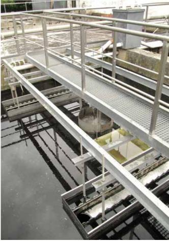
Fig. 4.270: Vertical settling tank (taken from: VHZ-DIS, 2021)
