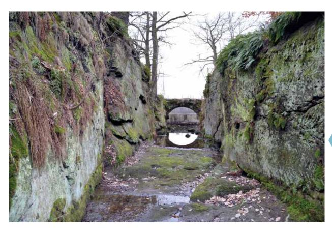
Fig. 4.91: Stvolínky, Dolanský Pond – a rock gulley of the safety spillway; in the background a bridge in the dam route. Photograph by Miroslav Kolka, 2016.
