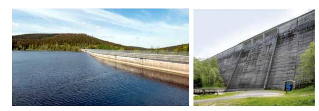
Fig. 4.43: The Fláje dam (1951–1963) – buttress dam. Photograph by Viktor Mácha, 2020.
