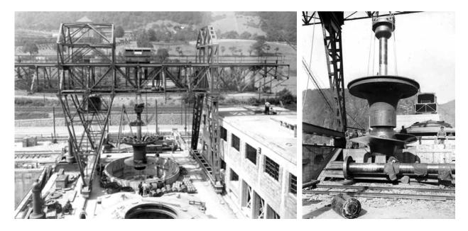
Fig. 4.200: Střekov HPP – a machine set with a vertical Kaplan turbine – installation of a runner (taken from: the Povodí Labe, s.p. [Elbe River Basin] archive).
