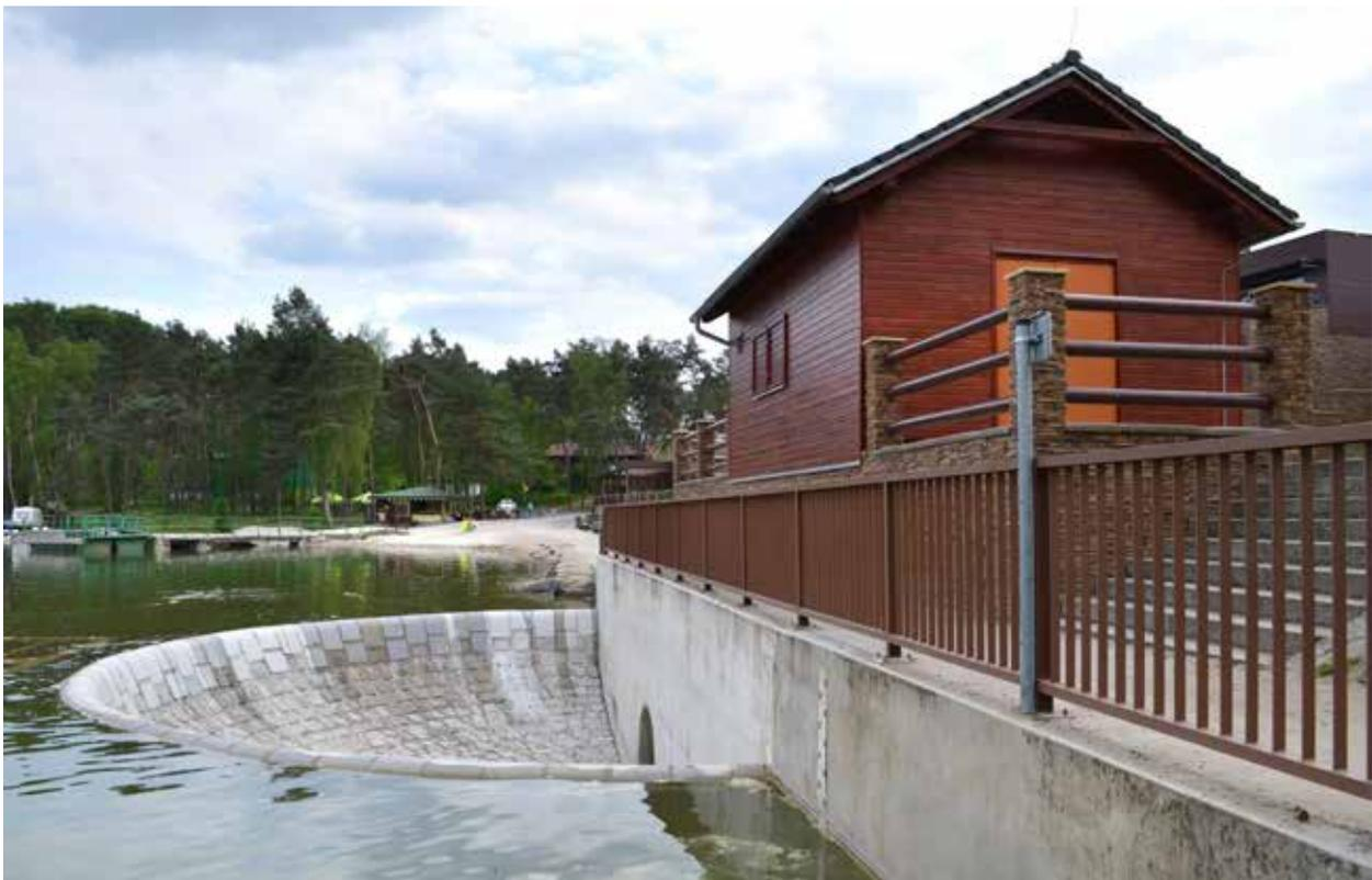
Fig. 4.55: Mácha Lake (1366) – straight earthfill dam from local materials, detail of fountain safety spillway. Photograph by Miroslav Kolka, 2016.
