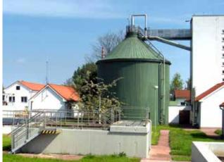
Fig. 4.280: Sludge handling and disposal within a WWTP – sludge-digestion tanks and biogas collection (taken from: the TGM WRI archive).
