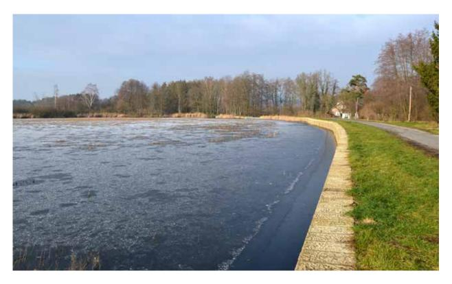
Fig. 4.75: Holany, Holanský Pond – a concave shape of a dam with a restored upstream wall from sandstone blocks. Photograph by Miroslav Kolka, 2018.
