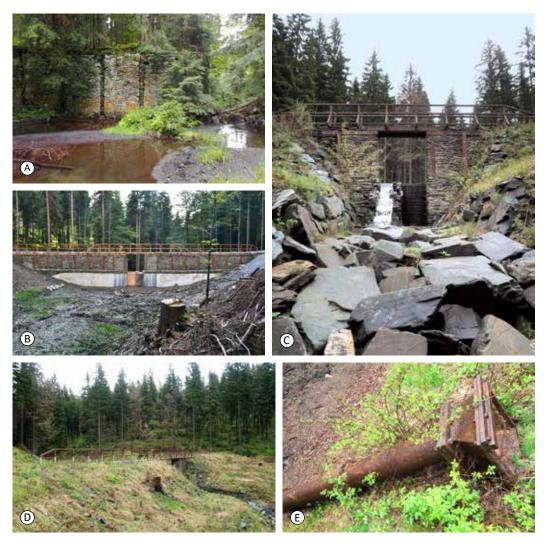
Fig. 5.309: Žďárský Potok, renewal of the splash dam on Splavský Brook: (A) remnants of the original dam (taken from: Rymarovsko.cz, 2021); (B) repaired dam from the upstream side (taken from: Rymarovsko.cz, 2021); (C) middle part of the dam with the flow section; (D) overall view of the dam from the downstream side; (E) original outlet piping. Photograph (C), (D) and (E) by Martin Caletka, 2021.
