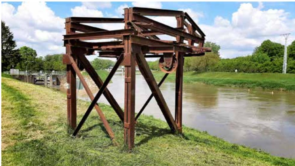
Fig. 4.111: Remnants of a boat funicular lift for crossing of the Baťa Canal with the Morava River near Vnorovy. Photograph from the TGM WRI archive, 2012.
