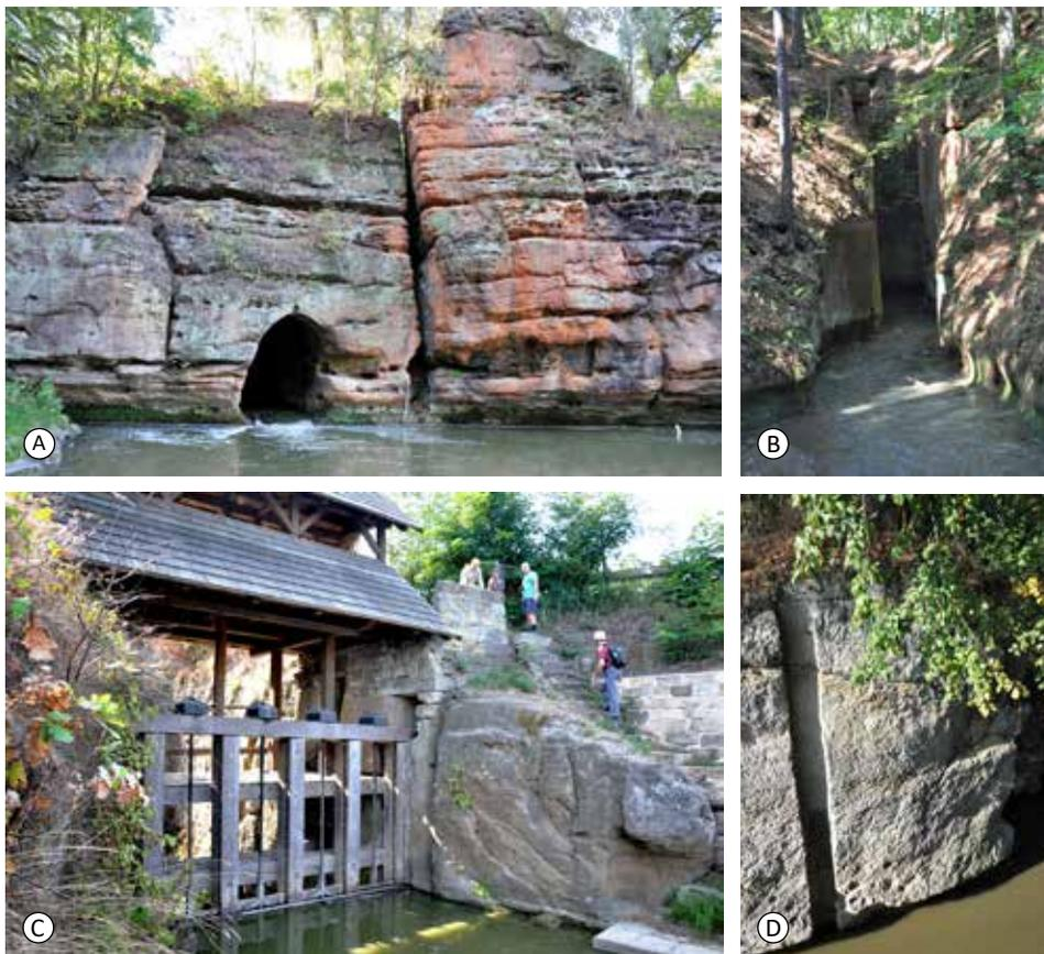
Fig. 4.114: Building material of water canals – sandstone: (A) and (B) Ploučnice gulley, artificial shortening of the watercourse by a tunnel and an open trough; (C) the siting of the structure with sluice gates directly into the sandstone block; (D) the detail of the groove for temporary flashboard cut in sandstone. Photograph by David Honek, 2019.
