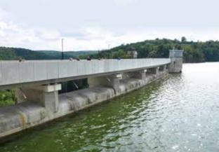
Fig. 4.38: The Vranov dam (1930–1934) – example of a concrete dam and uncontrolled crown spillway (on the right). Photograph by Michaela Ryšková, 2020.
