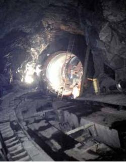
Fig. 4.175: Dlouhé stráně PSHPP – positioning of steel armour into the inlet gallery of turbines (taken from: Höll, 1997).
