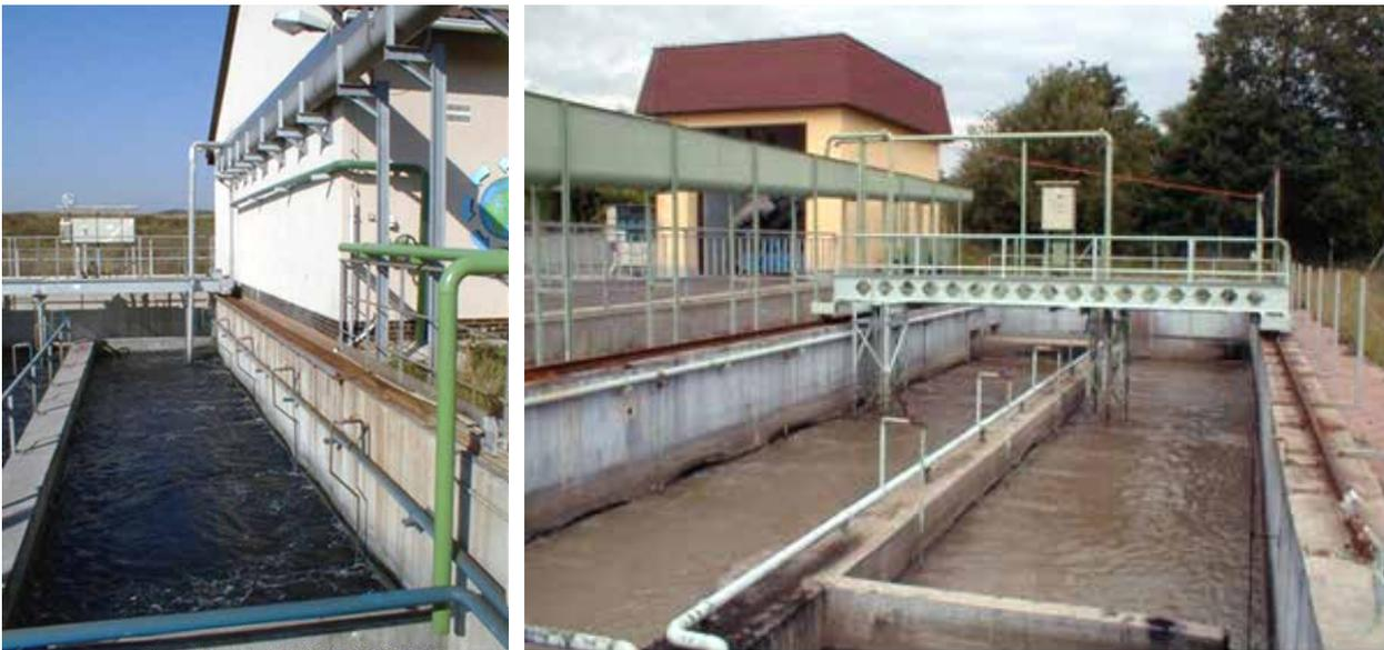
Fig. 4.265: Horizontal chamber sand trap (taken from: the TGM WRI archive).
