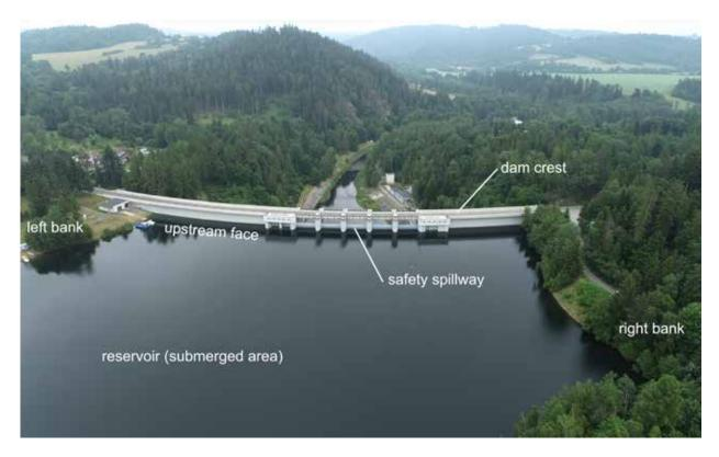
Fig. 4.26: Definitions of basic terms – the Kružberk dam (1948–1955). Photograph by Radek Bachan, 2021.
