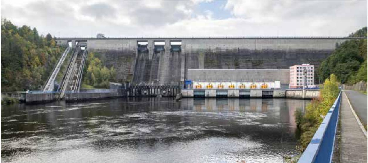
Fig. 4.39: The Orlik dam (1954–1963) – concrete gravity dam. Photograph by Viktor Mácha, 2021.
