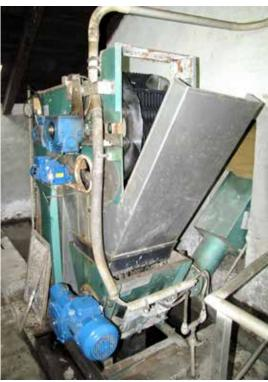
Fig. 4.263: Fine screen – machine-raked. Photograph by Miloš Rozkošný, 2021.
