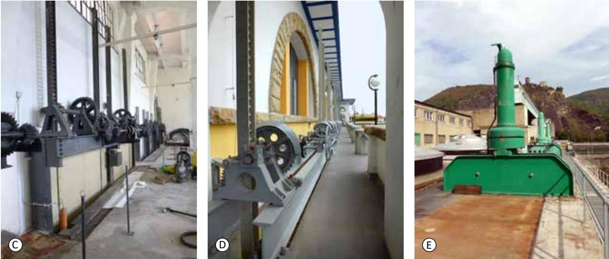
Fig. 4.163: Slide gates and cleaning machines on weir inlets of a small hydroelectric power plant: (A) and (D) Miřejovice SHPP. Photograph by Brno University of Technology, Faculty of Civil Engineering, 2014; (B) Kroměříž SHPP. Photograph by Miloš Matěj, 2016); (C) Háj SHPP near Třeština. Photograph by Michaela Ryšková, 2018; (E) Střekov HPP. Photograph by Michaela Ryšková, 2015.
