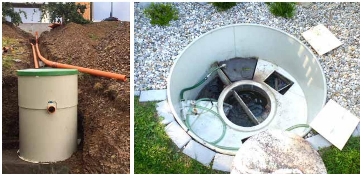
Fig. 4.281: Examples of domestic wastewater treatment plants (on the left, taken from: the Ekočov, s.r.o. archive, on the right, Rozkošný, 2012).
