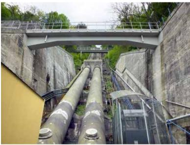
Fig. 4.178: Support block construction: (A) Diagram by Radka Račoch and Radek Bachan, 2021 (modified according to: Broža et al., 1990); (B) Štěchovice PSHPP – pressure pipeline with support and anchor blocks. Photograph by Brno University of Technology, Faculty of Civil Engineering, 2019.
