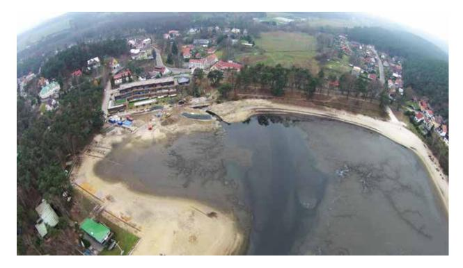
Fig. 4.74: Doksy – Staré Splavy, Mácha Lake – In the left part of the picture, a straight dam of a pond which consists of an outcrop of a sandstone bedrock with a basalt vein, in the middle part there is an outlet gully; state during the reconstruction of the outlet structure and the pond drawdown. Photograph by A. Kopecký, 2014.
