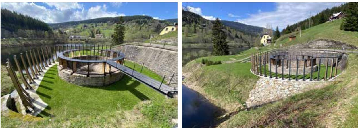
Fig. 4.53: The Labská dam (1910–1916) – masonry gravity dam, shaft safety spillway which was being reconstructed in 2017–2019. Photograph by Radka Račoch, 2021.
