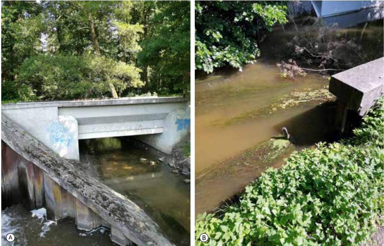
Fig. 4.116: The Semínský aqueduct on the Opatovice Canal. (A) state after reconstruction; (B) remains of old wooden elements. Photograph by David Honek, 2020.
