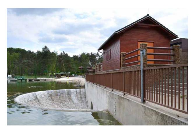
Fig. 4.55: Mácha Lake (1366) – straight earthfill dam from local materials, detail of fountain safety spillway. Photograph by Miroslav Kolka, 2016.
