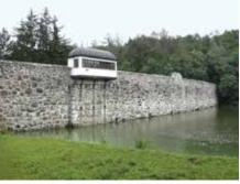
Fig. 3.7: The Jevišovice dam (1884–1896) is one of the two oldest masonry-built dams in the Czech Republic, dating from 1884–1896. The authenticity of form has been disrupted by modifications to the crest of the dam and the addition of an engine room containing the control mechanisms for the bottom outlets. Historical postcard, collection of Michaela Ryšková. Photograph by Michaela Ryšková, 2020.
