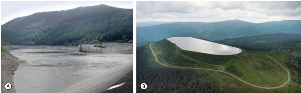
Fig. 3.21: Dlouhé stráně PSHP: (A) lower reservoir; (B) upper reservoir; an example of upper and lower reservoirs with controversial landscape/urbanistic value and a substantial impact on the appearance of the location. The upper reservoir has had a major impact on the panorama of the High Jeseníky mountains due to the removal of the hill's original summit, which has been levelled. Photograph by (A) David Honek, 2019, (B) by Shutterstock, 2021.
