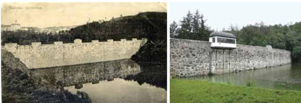
*Fig. 3.7: The Jevišovice dam (1884–1896) is one of the two oldest masonry-built dams in the Czech Republic, dating from 1884–1896. The authenticity of form has been disrupted by modifications to the crest of the dam and the addition of an engine room containing the control mechanisms for the bottom outlets. Historical postcard, collection of Michaela Ryšková. Photograph by Michaela Ryšková, 2020.*
