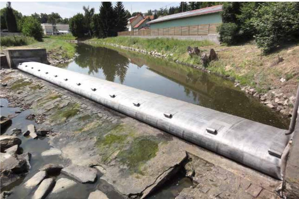
Fig. 4.136: An inflatable weir in Jihlava. Photograph from the Brno University of Technology archive, 2013.
