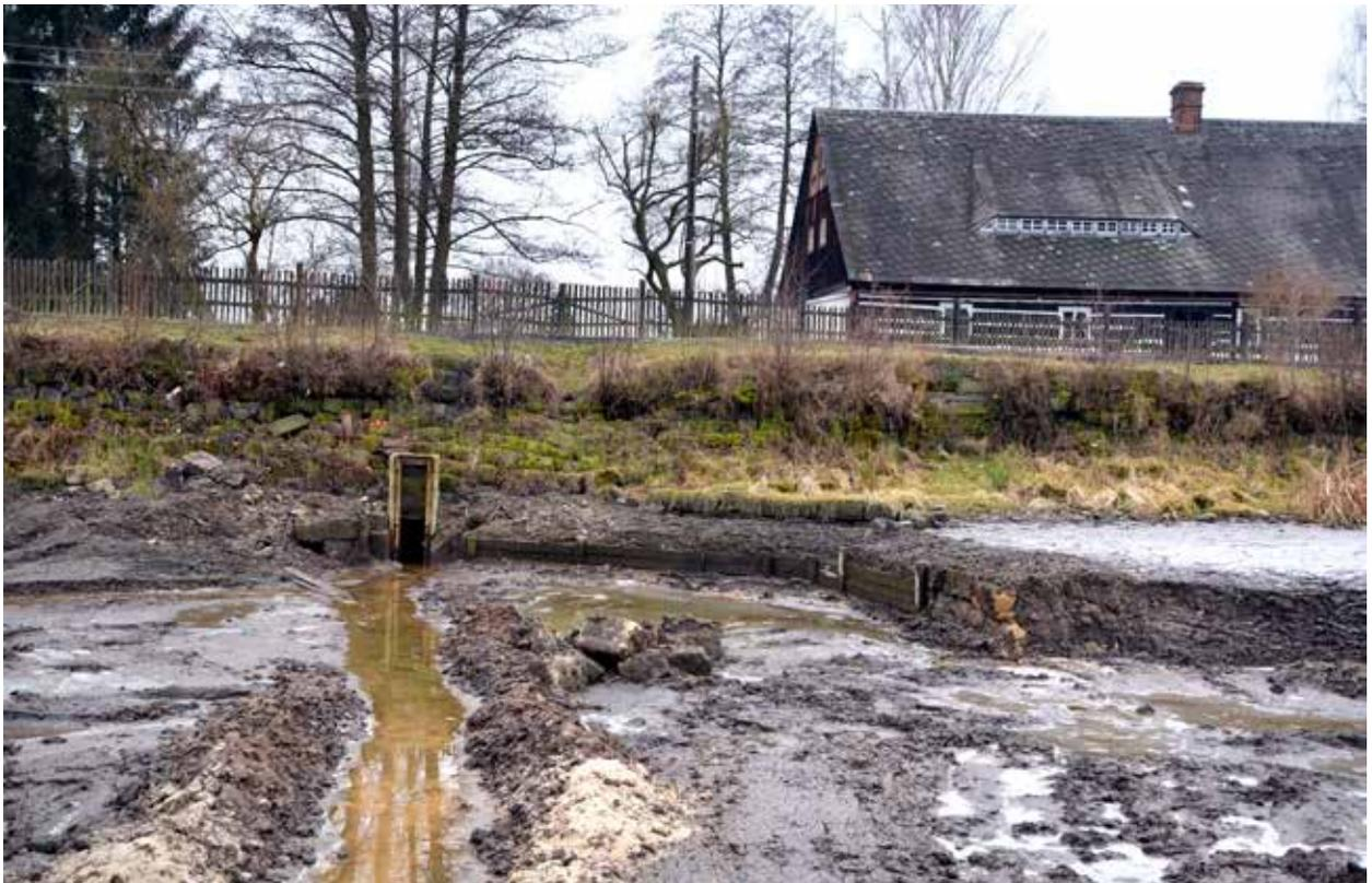
*Fig. 4.88: Markvartice near Jablonné v Podještědí, Markvartický Pond – the bottom outlet of the idle discharge with a monk outlet, upstream face with typical revetment from sandstone blocks; state after the pond drawdown. Photograph by Miroslav Kolka, 2014.*
