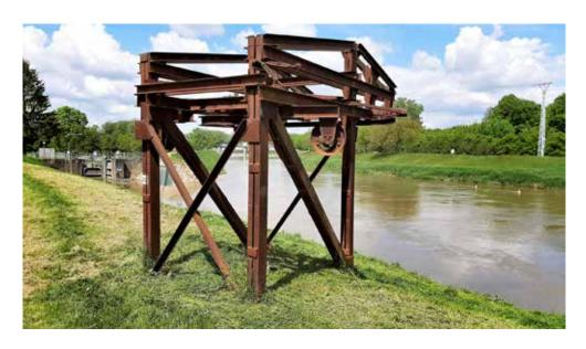
Fig. 4.111: Remnants of a boat funicular lift for crossing of the Baťa Canal with the Morava River near Vnorovy. Photograph from the TGM WRI archive, 2012.
