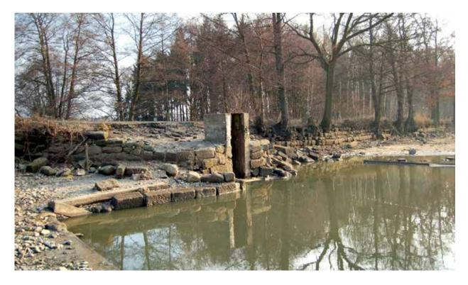
Fig. 4.79: Holany, Jílovka Pond – construction of the dam with the revetment of the upstream face from sandstone masonry, a part of the revetment in connection with the main outlet and the fishing ground. Photograph by Miroslav Kolka, 2018.
