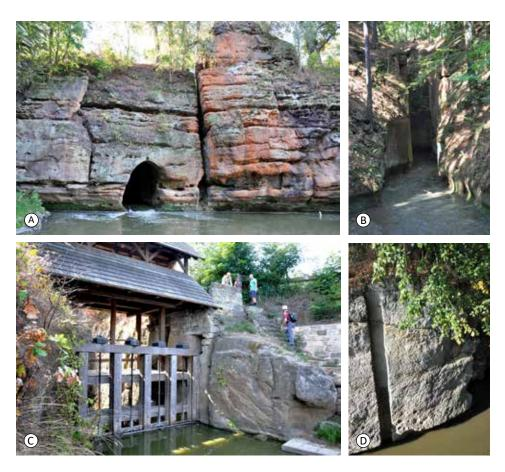
Fig. 4.114: Building material of water canals – sandstone: (A) and (B) Ploučnice gulley, artificial shortening of the watercourse by a tunnel and an open trough; (C) the siting of the structure with sluice gates directly into the sandstone block; (D) the detail of the groove for temporary flashboard cut in sandstone. Photograph by David Honek, 2019.
