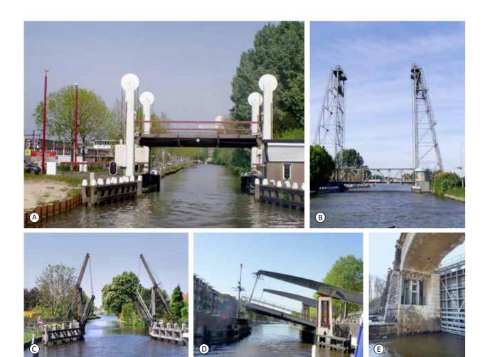
Fig. 4.107: Moveable bridges of various structures: (A) and (B) with counterweight, raised with a road in the horizontal position; (C), (D) bascule bridges; (E) hydraulic bridge on the reconstructed lock Hořín. Photograph (A)–(D) by Vít Forejtník, 2007 (Netherlands); Photograph (E) by Otakar Hrdlička, 2021.
