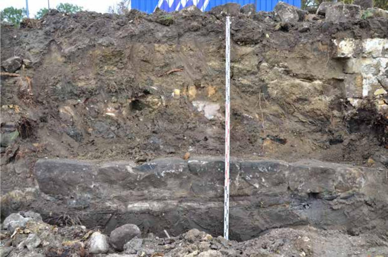
*Fig. 4.78: Holany, Holanský Pond – construction of the dam with the revetment of the upstream face, the sandstone masonry is founded on the beam grid from the beginning of the 16th century. Photograph by Miroslav Kolka, 2018.*
