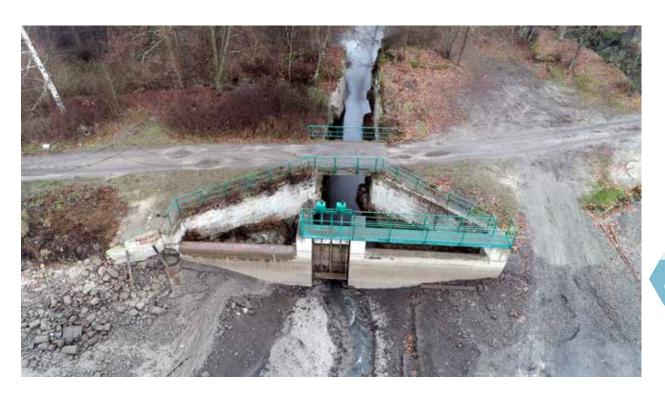
Fig. 4.80: Holany, Holanský Pond – the main outlet with a discharge to the sandstone rock gulley. Photograph by J. Vidman, 2018.
