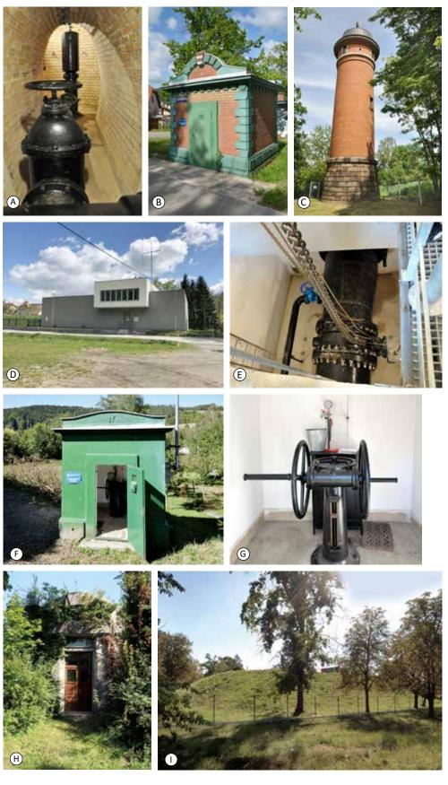
Fig. 4.255: The 1st Březová aqueduct – selected parts: (A) well machinery equipment; (B) slide chamber in Blansko; (C) Letovice relief tower; (D) Březová nad Svitavou ground water tank; (E) pipeline; (F) Březová nad Svitavou gate valve chamber; (G) gate valve chamber control equipment; (H) entry into Holé Hory II ground water tank and (I) Holé Hory II ground water tank. Photograph by David Honek, Miriam Dzuráková, 2019 a 2020.
