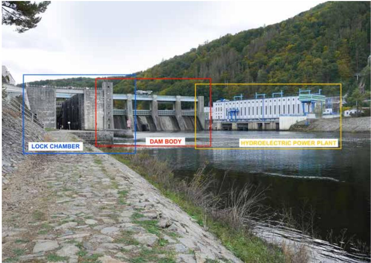
*Fig. 4.59: The Štěchovice HS (1937–1945) – concrete gravity dam. Example of a functional complex – dam + lock chamber + hydroelectric power plant. Photograph by Michaela Ryšková, 2020.*
