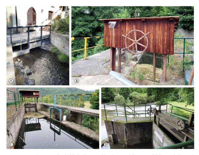
Fig. 4.118: Control structures details: (A) Chrudim – wood, hand-operated sluice gates; (B) the Weisshuhn Canal, an originally hand-operated sluice gate converted into electrically-powered; (C) the same place, right-bank residual outflow operated hydraulically; (D) mechanism for manual control of sluice gates from the side. Photograph by Radka Račoch, 2021.
