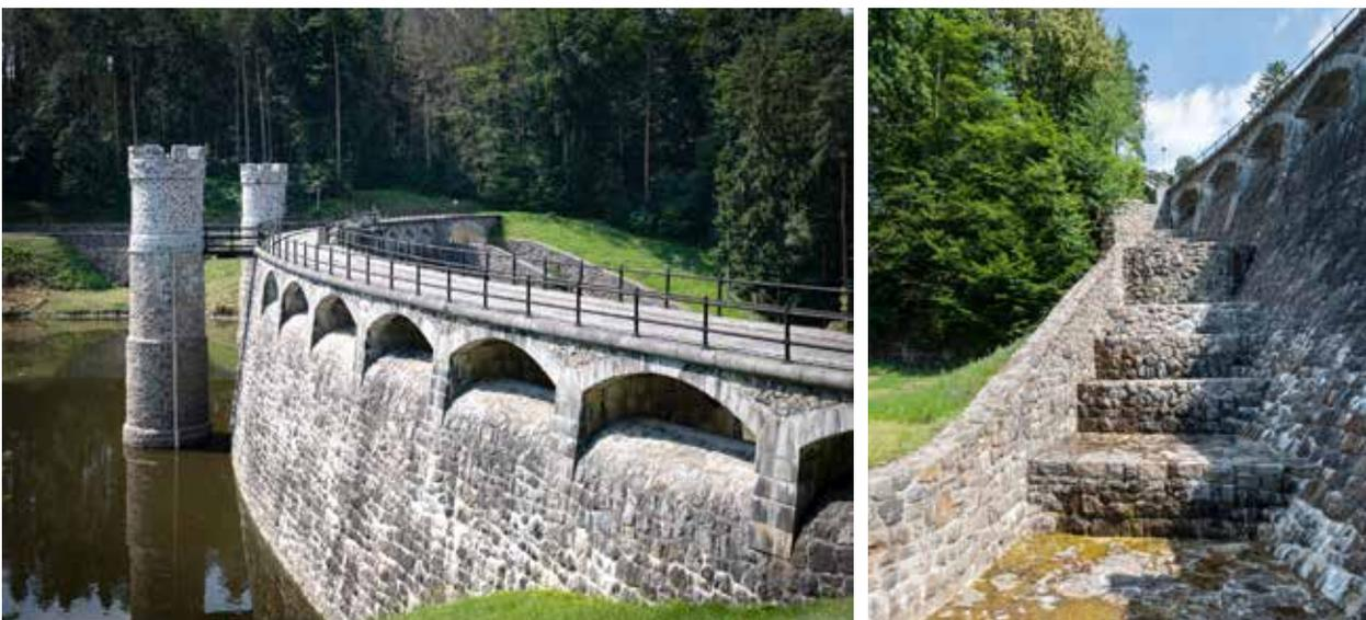
*Fig. 4.36: The Pařížov dam (1909–1913) – On the left, the view on the crown safety spillway from the upstream side. On the right, the view from the downstream side on the crown spillway cascade. Photograph by Viktor Mácha, 2020.*
