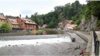
Fig. 4.135: Sector weir. Diagram by Radka Račoch and Michaela Mrvová, 2021 (modified according to: Jermář, 1956). On the right, a sector weir on the Vltava River in Český Krumlov. Photograph from the Brno University of Technology archive, 2019.
