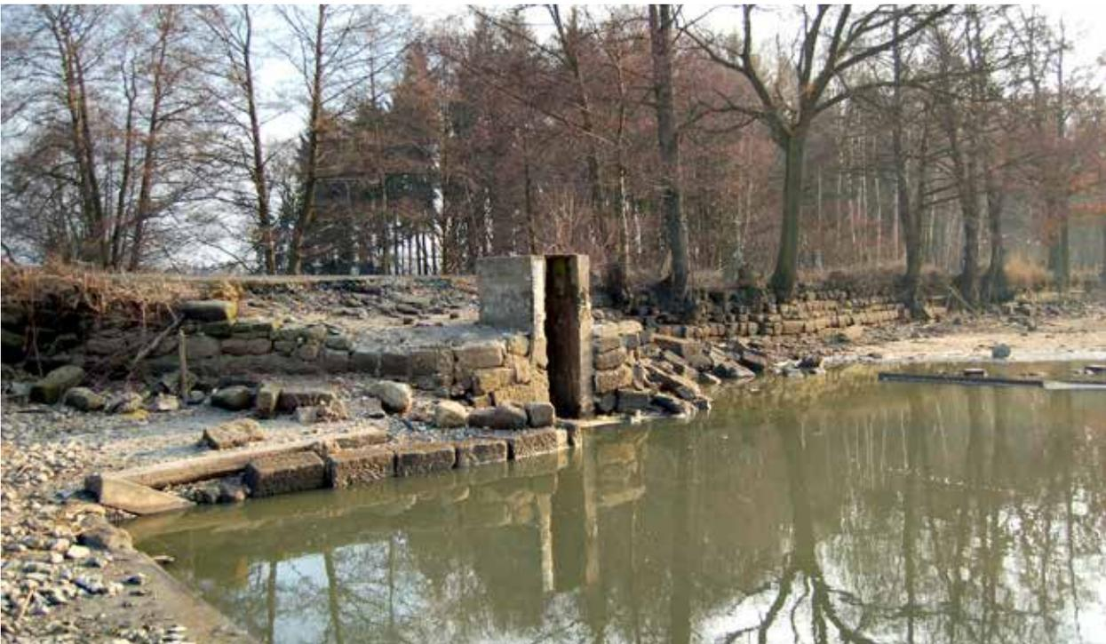
*Fig. 4.79: Holany, Jílovka Pond – construction of the dam with the revetment of the upstream face from sandstone masonry, a part of the revetment in connection with the main outlet and the fishing ground. Photograph by Miroslav Kolka, 2018.*
