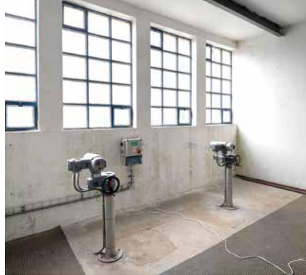
Fig. 4.48: The Vrchlice dam (1966–1970) – arch dam. On the left, operational Howell Bunger valve of bottom outlets. On the right, control equipment of Howell Bunger valves. Photograph by Viktor Mácha, 2020.
