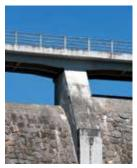
Fig. 4.50: The Pastviny dam (1933–1938) – masonry gravity dam. The last masonry-built dam in the Czech Republic to this day. In the pictures, there is an uncontrolled crown spillway with six bays having different overflow edge levels. Water is diverted through a chute into a stilling basin which is shut by a stepped sill. Photograph by Viktor Mácha, 2020.
