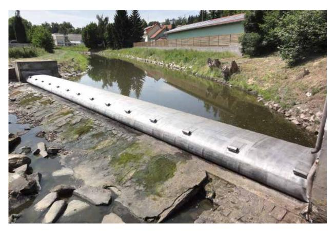
Fig. 4.136: An inflatable weir in Jihlava. Photograph from the Brno University of Technology archive, 2013.
