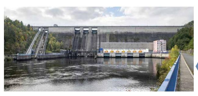
Fig. 4.39: The Orlík dam (1954–1963) – concrete gravity dam. Photograph by Viktor Mácha, 2021.
