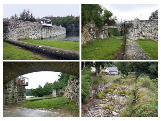
Fig. 4.52: The Jevišovice dam (1884–1896) – masonry gravity dam. Top left, overflow edge of an uncontrolled side safety spillway. Top right, overflow edge and drop structure. Bottom left, view into the drop structure from under the bridge. Bottom right, the chute. Photograph by Michaela Ryšková, 2020.
