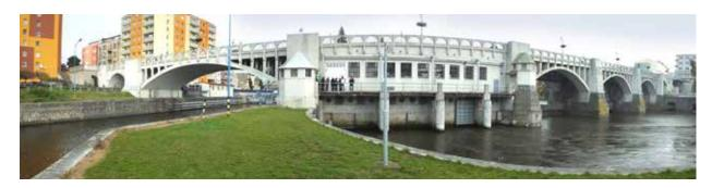
Fig. 4.155: Kolín SHPP – a view from the area downstream of the weir of the machine room and the outlet part of the small hydroelectric power plant (on the left) and three sections of the roller drum weir (on the right). Photograph by Brno University of Technology, Faculty of Civil Engineering, 2014.
