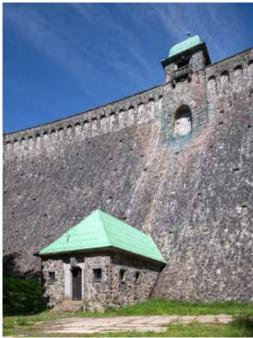
Fig. 4.32: The Janov dam (1911–1914) – an example of a masonry dam. Photograph by Viktor Mácha, 2020.
