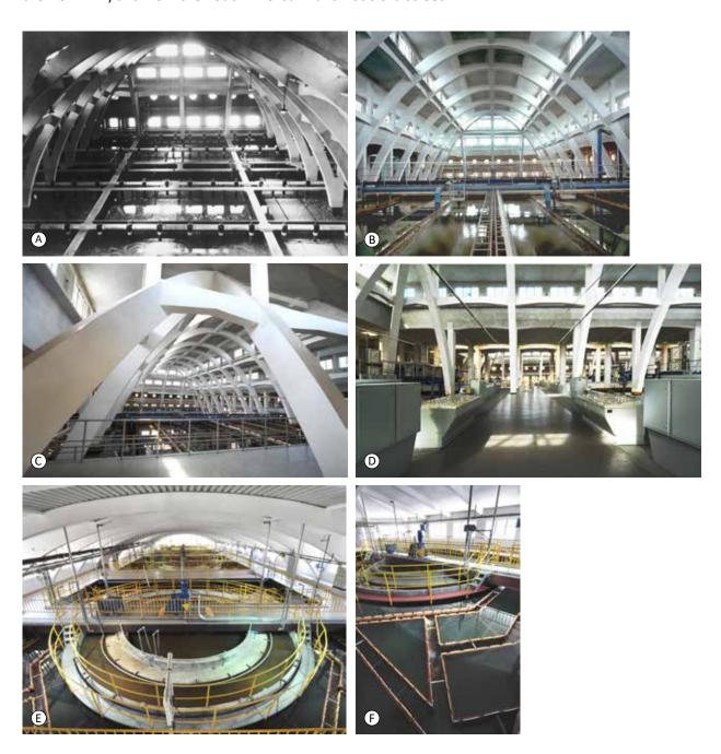
Fig. 4.257: Prague-Podolí water treatment plant (A) original filtration hall in the 1930s; (B) current filtration tanks; (C) and (D) view of the supporting arch system; (E) and (F) one of the clarifier halls. Photograph by the PVK archive and Jaroslav Beneš, 2018.
