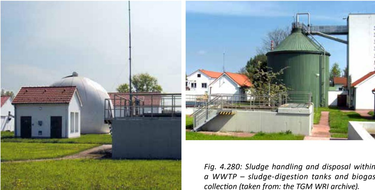
*Fig. 4.280: Sludge handling and disposal within a WWTP – sludge-digestion tanks and biogas collection (taken from: the TGM WRI archive).*
