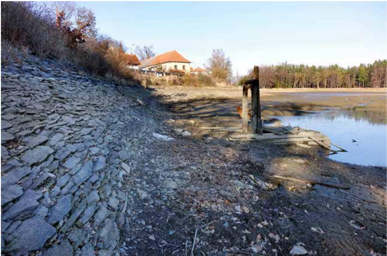
*Fig. 4.77: Stone riprap of the upstream dam side of Zbýšovský Pond. Photograph by Jindřich Frajer, 2018.*
