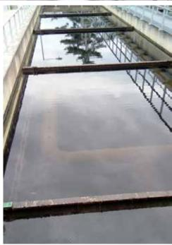
Fig. 4.267: Horizontal settling tank. Photograph by Miloš Rozkošný, 2021.
