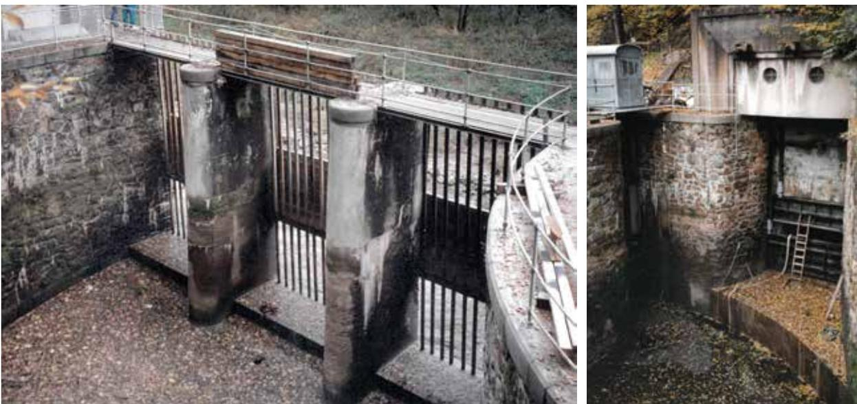
Fig. 4.167: Spálov derivation SHPP – inlet structure, state without water at the time of repair in 1998. Photograph by Brno University of Technology, Faculty of Civil Engineering, 1998.
