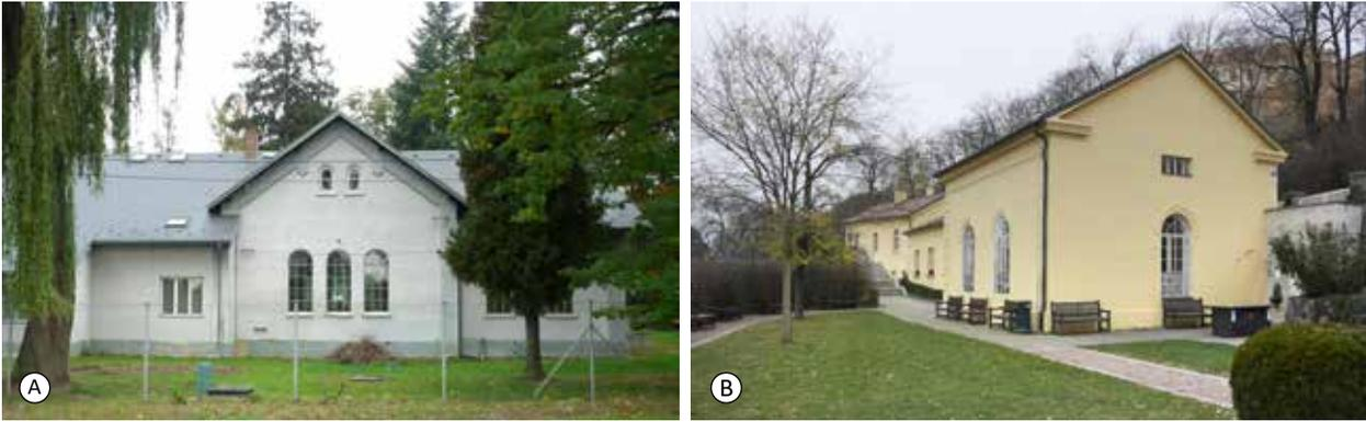
*Fig. 3.10: Former pumping stations: (A) Opava, the appearance of this former steam-powered pumping station is characteristic of this type of building. It was a single-floor structure with a gable roof and windows incorporating semicircular upper sections. Photograph by Alena Borovcová; (B) Brno, former pumping station at Špilberk. Photograph by Michaela Ryšková, 2021.*
