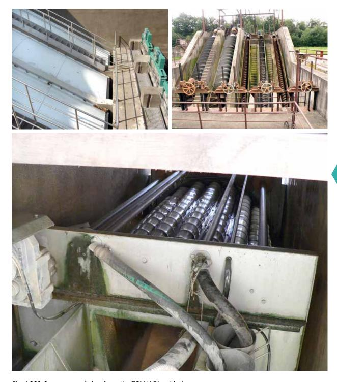
Fig. 4.266: Screw pumps (taken from: the TGM WRI archive).
