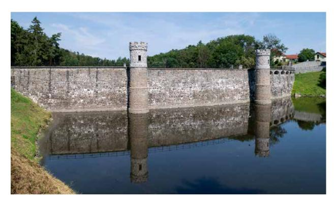
Fig. 4.33: The Pařížov dam (1909–1913) – control towers on the upstream side of the dam for the handling of inspection slide gate valves. Photograph by Viktor Mácha, 2020.
