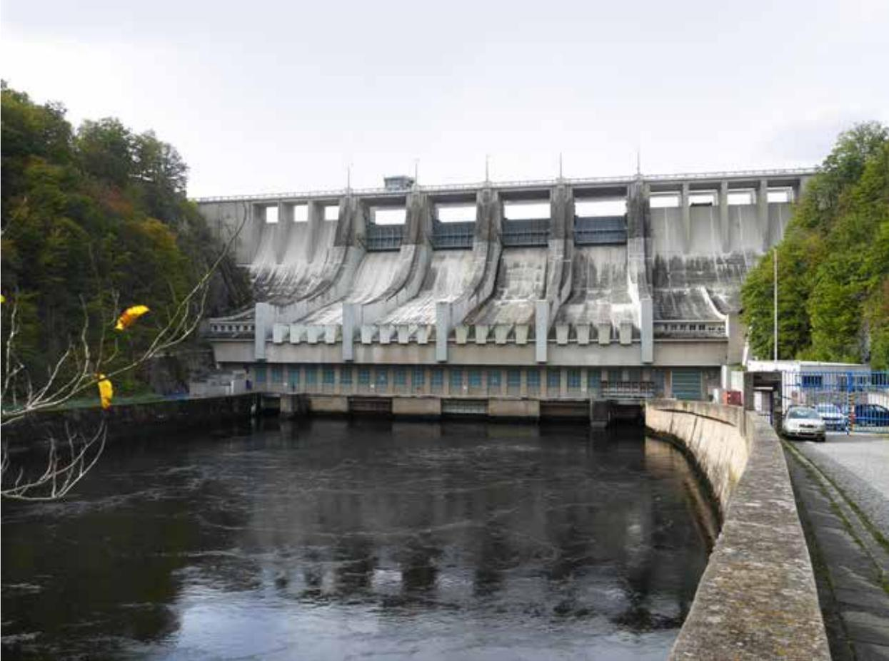
*Fig. 4.65: The Slapy dam (1949–1957) – concrete gravity dam, crown safety spillway with four sections controlled by a lifting gate. Photograph by Viktor Mácha, 2021.*
