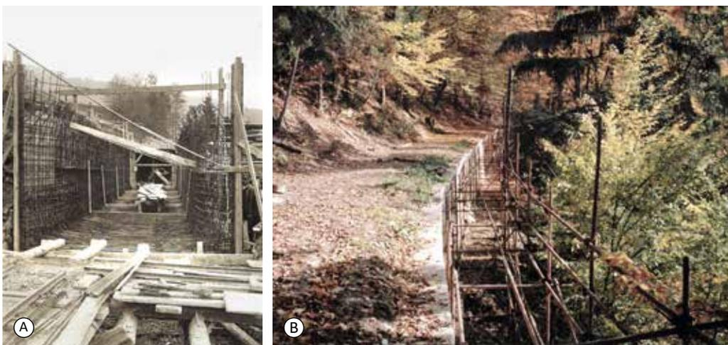
Fig. 4.173: Spálov SHPP – reinforced concrete supply channel: (A) reinforcement procedure in 1925. Taken from: VČE, 2000; (B) view from the channel ceiling in 1998 during reconstruction. On the right, photograph by Brno University of Technology, Faculty of Civil Engineering, 1998.
