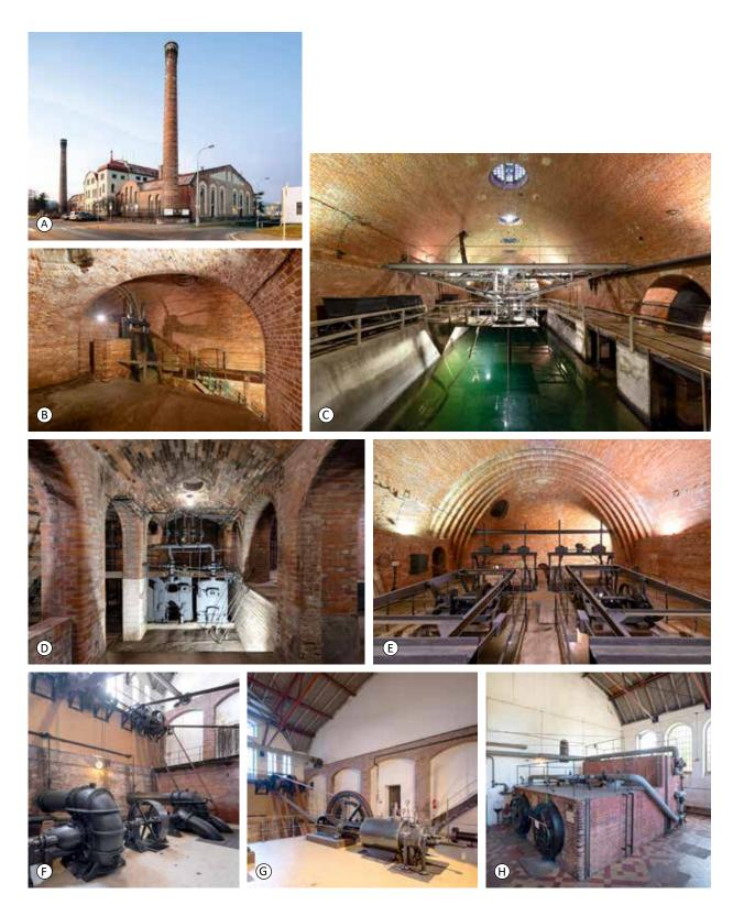
Fig. 4.293: Prague-Bubeneč. Old wastewater treatment plant. Legend: (A) overall view; (B) sewer sluice gate; (C) sand trap; (D) boiler room and coal room for the production of hot water and heating (originally premises for lime water tanks); (E) screen; (F)–(G) steam engine machine room; (H) boiler room. Photograph by Viktor Mácha, 2019.
