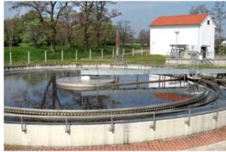
Fig. 4.268: Radial settling tank (taken from: the TGM WRI archive).
