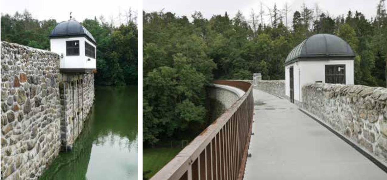
*Fig. 5.323: The Jevišovice dam – structure for handling bottom outlets. Photograph by Michaela Ryšková, 2020.*
