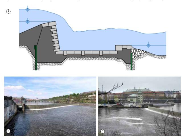
Fig. 4.125: (A) Masonry weir. Diagram by Radka Račoch and Radek Bachan, 2021 (modified according to: Průcha, 1980). (B–C) The Helmovský weir on the Vltava River with an Art Nouveau small hydroelectric power plant on the right bank. Photograph (B) Miriam Dzuráková, 2022, (C) Michaela Ryšková, 2022.
