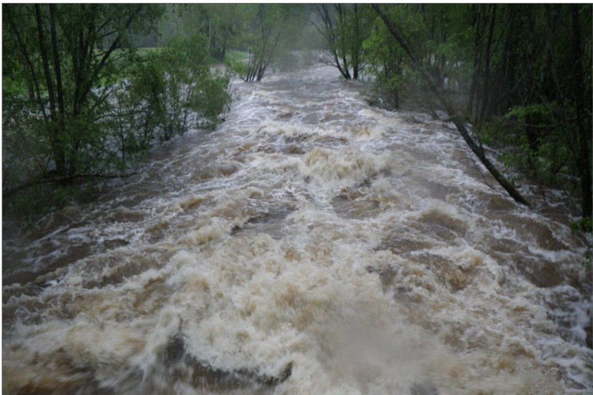
Fig. 178. Examples of problematic incidents at an RRF. A 'fifty-year flood' on the Blanice River in 2013. Photo: Ondřej Spisar.
