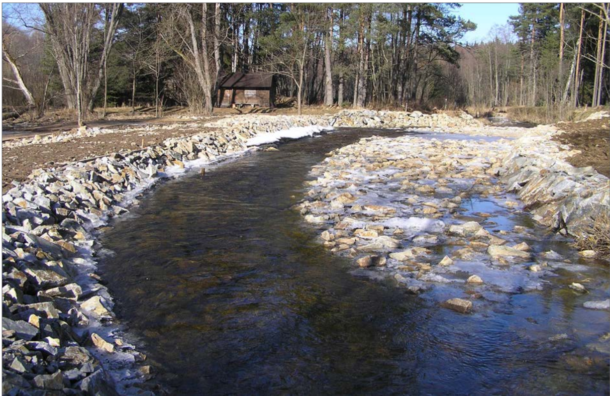
Fig. 206. Loose quarry stone meander reinforcement, created for the necessary stabilization of the bank above the transverse stage irrigating the side branch at the Spálenec RRF.
