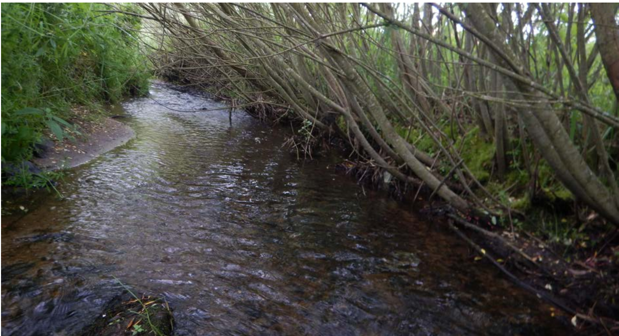
Fig. 260. General view of Zbytinský potok stream at water level on the longest growing fascine bundles with gravel after ten years (2016).
