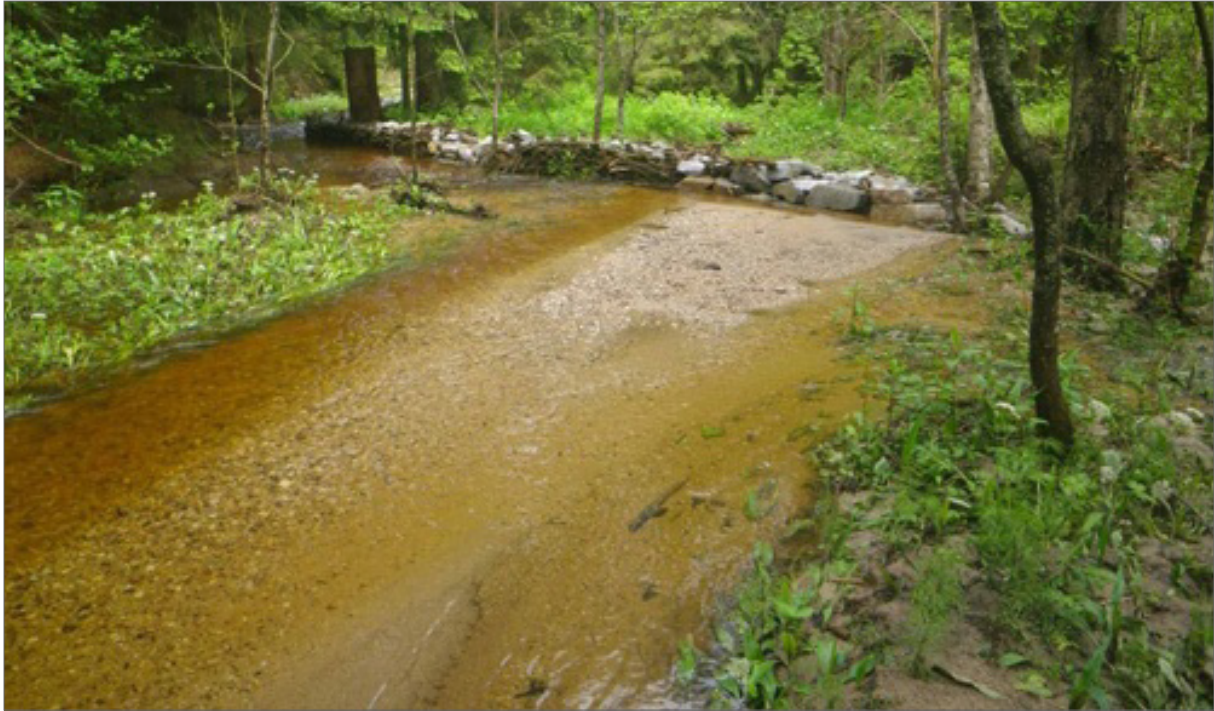
Fig. 191. Measures on Luční potok stream in the Zlatý potok stream catchment after the high water level has fallen – coarse sand is deposited in the river channel, finer sediment on the sides (not visible).
