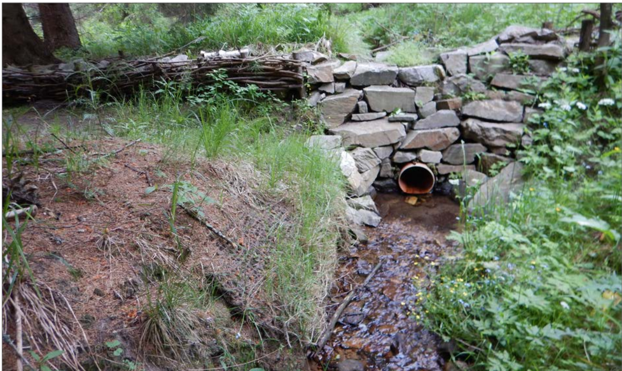
Fig. 192. Similar location to Fig. 189 after the passage of several floods (followed by the cleaning of the pipe surroundings) and the return of dense vegetation.
