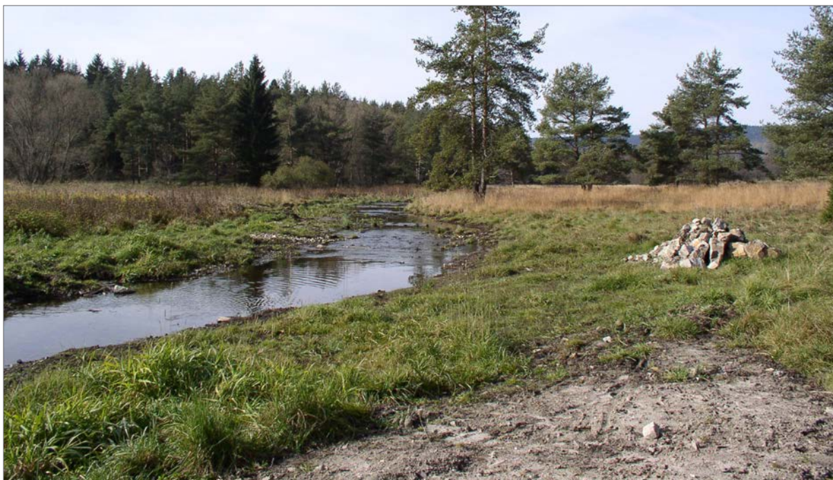
Fig. 187. A free spill into the tall grass floodplain meadow with Phalaris arundinacea and Filipendula ulmaria following after the sedimentation pool on Zbytinský potok stream (Fig. 186). The pool caught the sand and the spill caught part of the fine clay particles. Sediment from the pool had to be repeatedly removed using an excavator.
