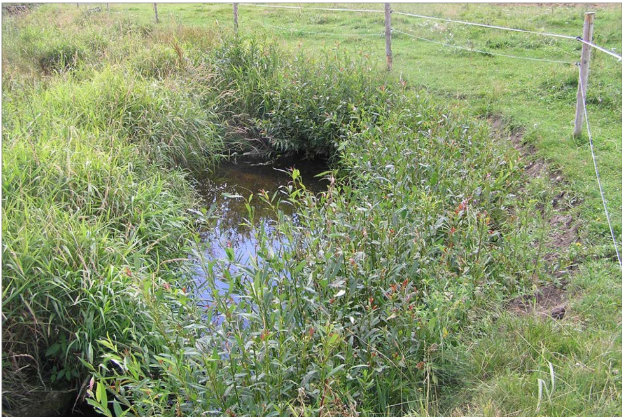
Fig. 258. The same set of two fascine bundles remediating a 150 cm high erosion wall after one vegetation season, 2007 (vegetation near the fencing was partially browsed by cows, the height of the vegetation up to 80 cm).
