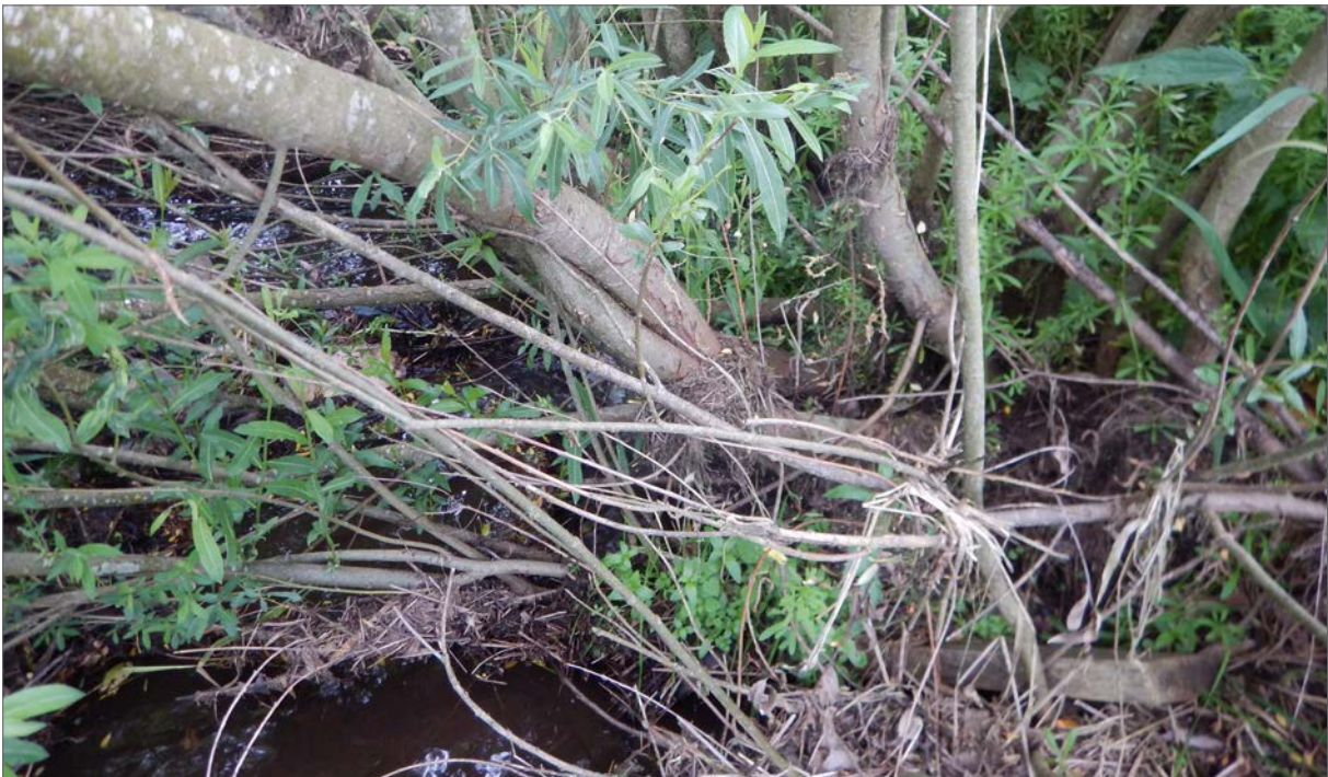
Fig. 203. Detail of a site where a fascine bundle was placed – the erosion control function was taken over by the dense riparian stand of rooted willow rods ( Salix fragilis ).
