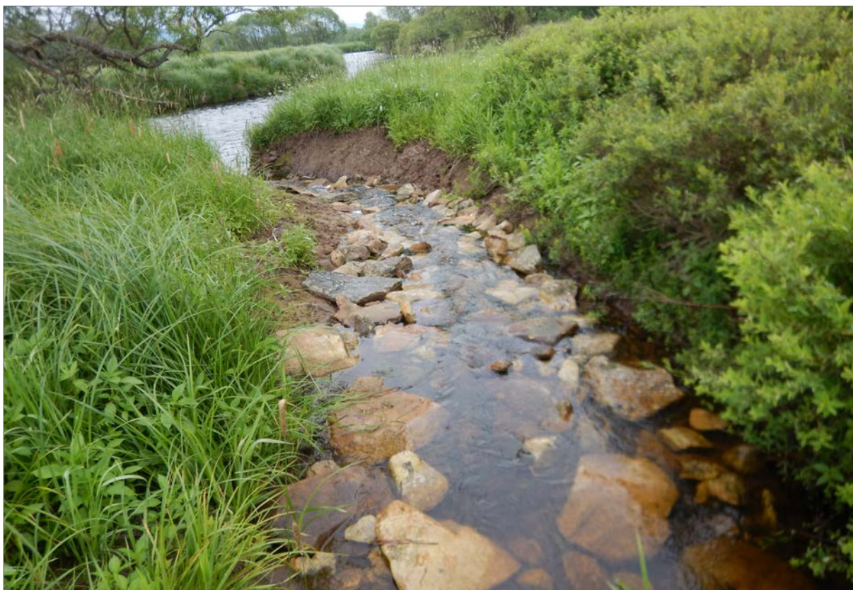
Fig. 170. The steep mouth of Žlebský potok stream into the Teplá Vltava River. The channel has been modelled and reinforced with stones, unlike the flat floodplain where there was room for the water to spontaneously form the channel.
