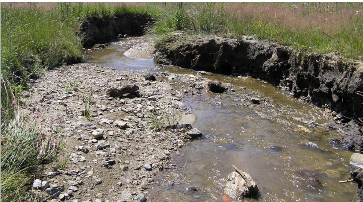
Fig. 168. Massive erosion processes started by increased flow rates during springtime snowmelt on the restored Zbytinský potok stream, causing the erosion and transportation of fine grain material, sand, and gravel into the main flow of the Blanice River.
