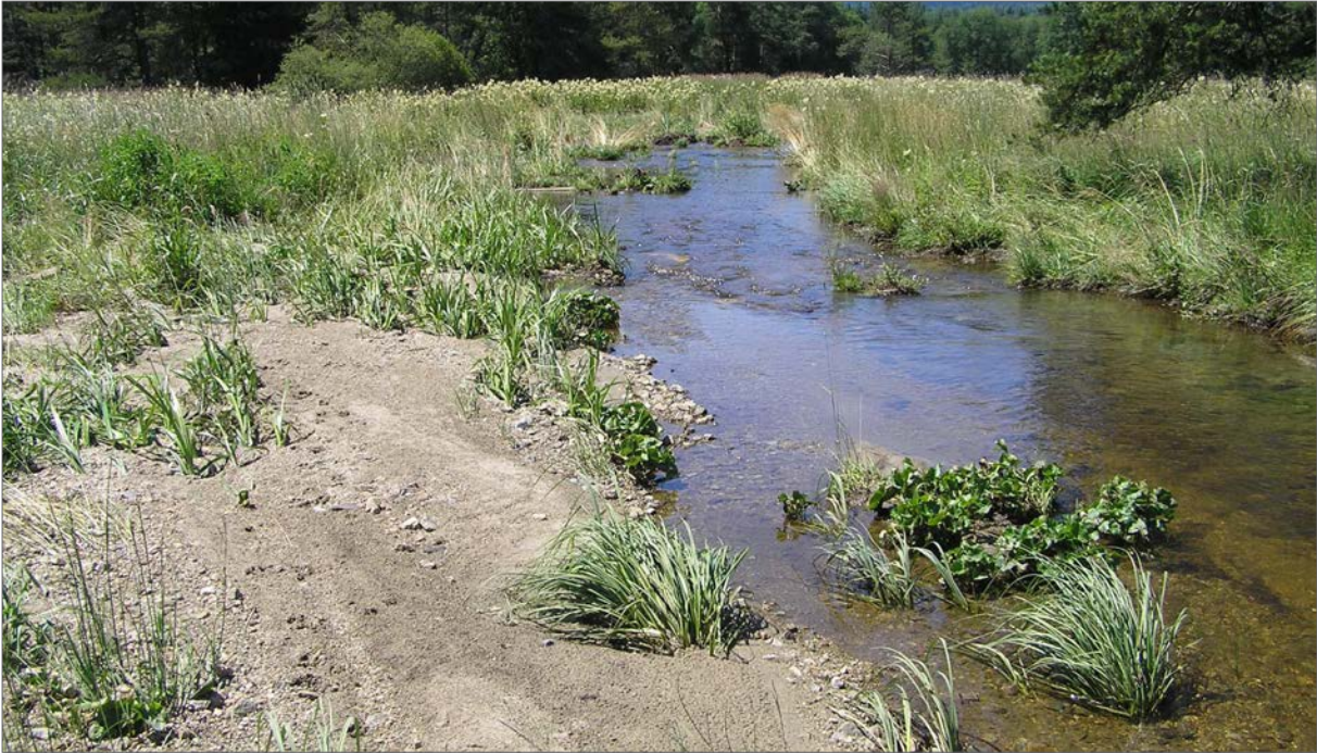
Fig. 182. Trapping eroded sediments in sedimentation pools. Sedimentation pool below the village of Zbytiny – a large amount of sand is apparent in the left of the picture, trapped by the pool during increased flow; on the right side, the main stream flows into the tall grass floodplain meadow where fine sediments settle (photo from 2012).
