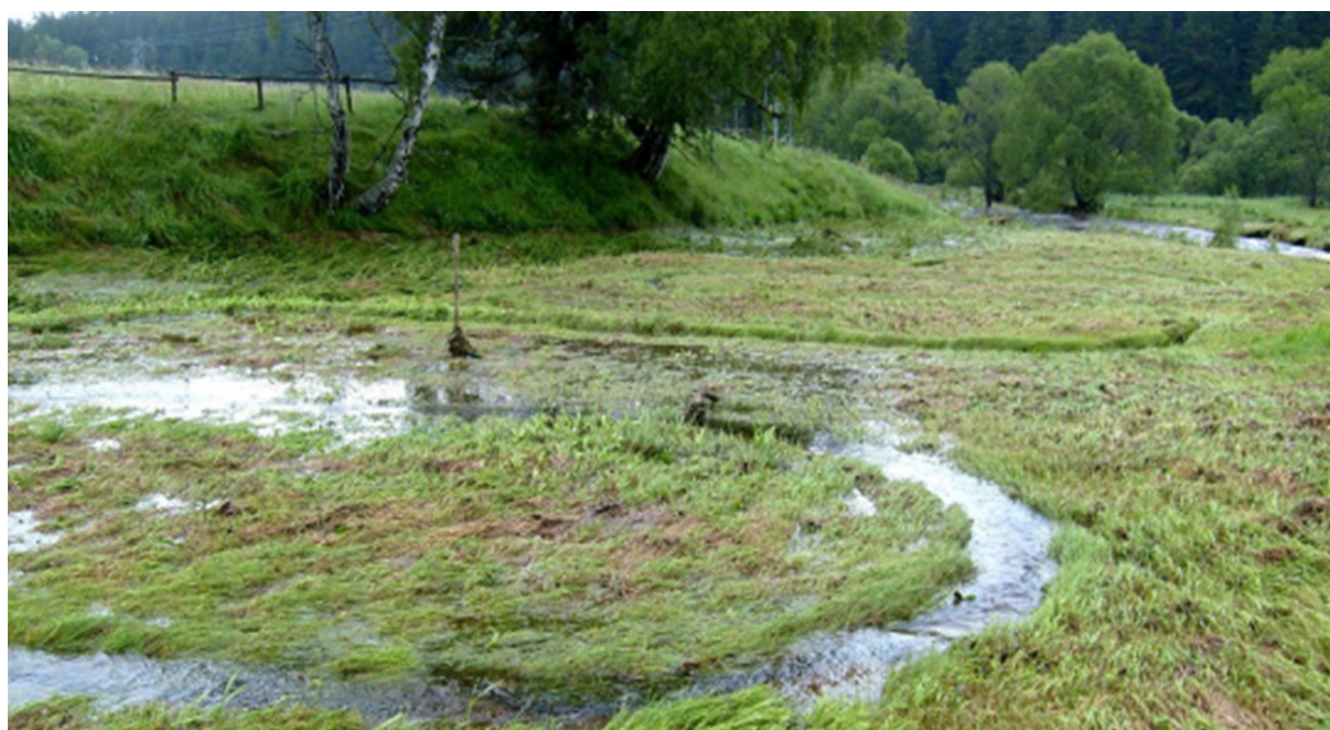
Fig. 36. RRF on Spálenecký potok stream in the Blanice River floodplain after 10-year floods. There was no mechanical damage of rills or sediment silting in the SRRF.
