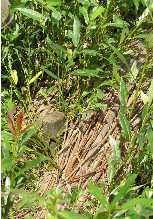
Fig. 259. Growing fascine bundles with gravel detail after one vegetation season, 2007 (fastening pole made of spruce log, bundles of wicker tied with burnt wire; they sprout densely and root from below).
