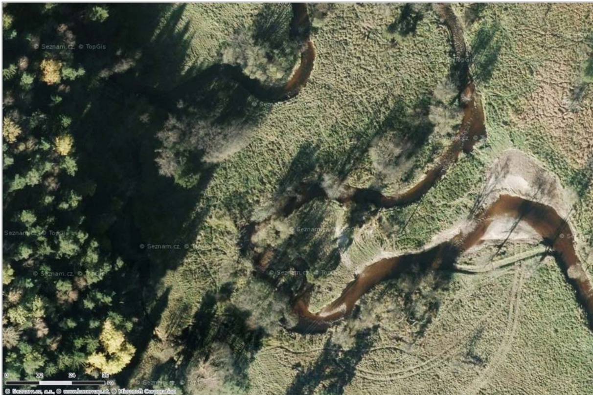
Fig. 210. Meander strengthening below the power transmission line on the main stream of the Blanice River – location and extent of the works. Source: Mapy.cz, © Seznam.cz, a. s., © TopGis, s. r. o.
