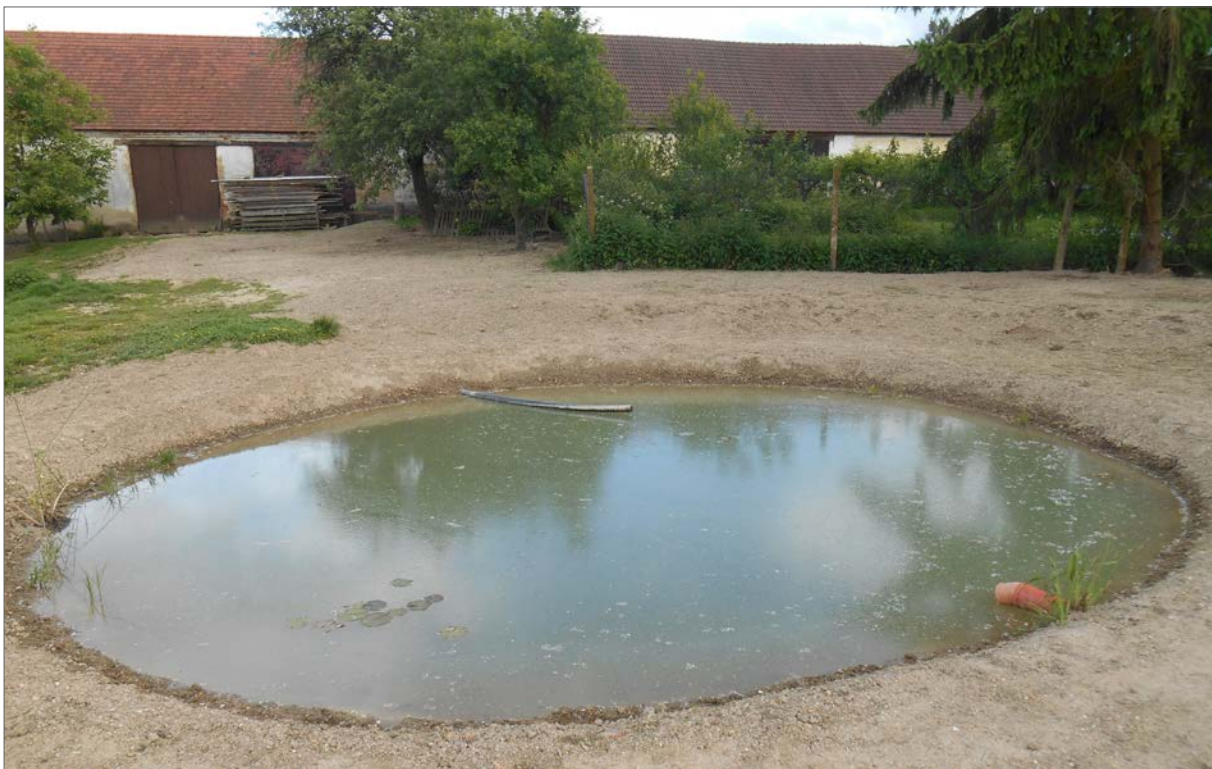
Fig. 112. A small post-treatment pond for five equivalent inhabitants next to a farmhouse in Malovice near Vodňany, adjacent to a domestic WWTP shortly after being built (a simple in-ground reservoir in argillaceous soil). The first of two low-loaded biological reservoirs.
