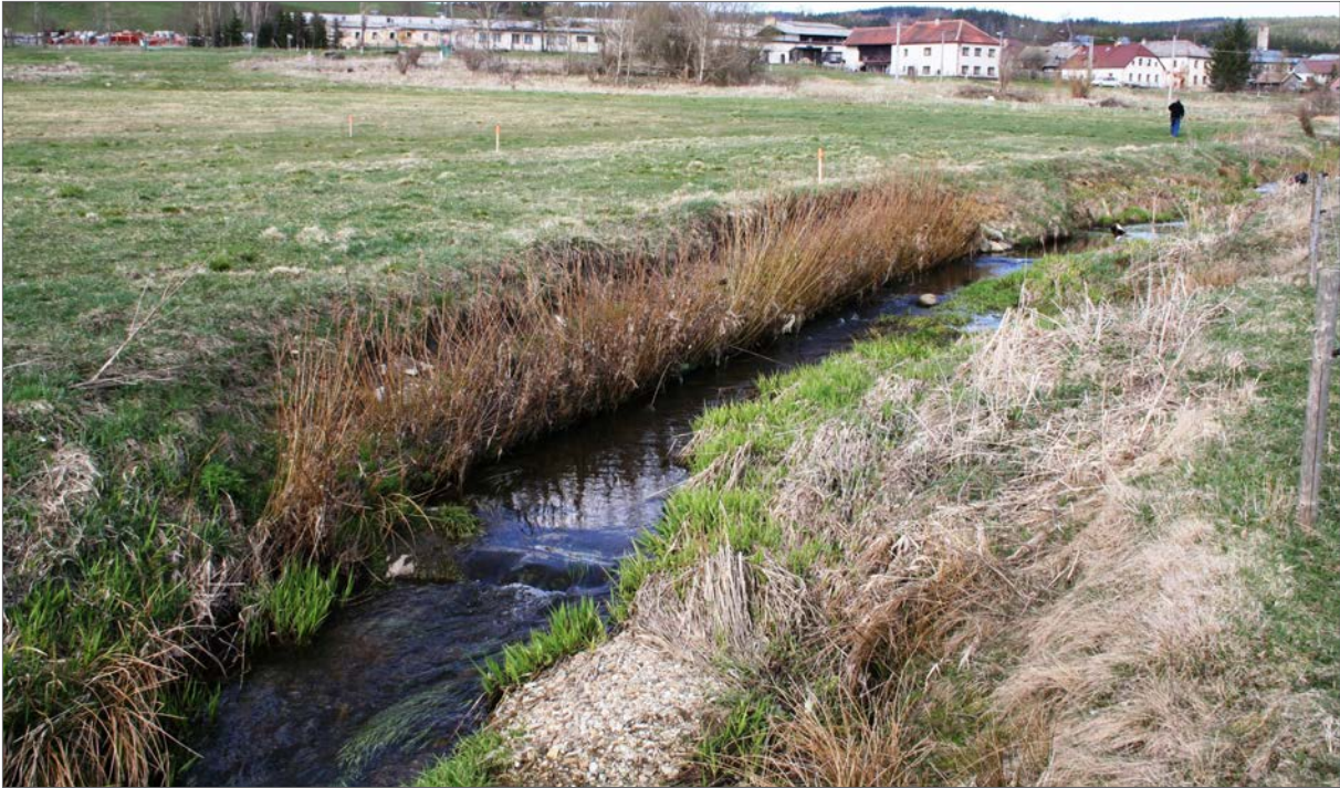
Fig. 196. Zbytinský potok stream in the village of Zbytiny – reinforcement of the eroded channel with a fascine bundle. Growth on the fascine bundle after the first growing season (for details, see Annex 14).
