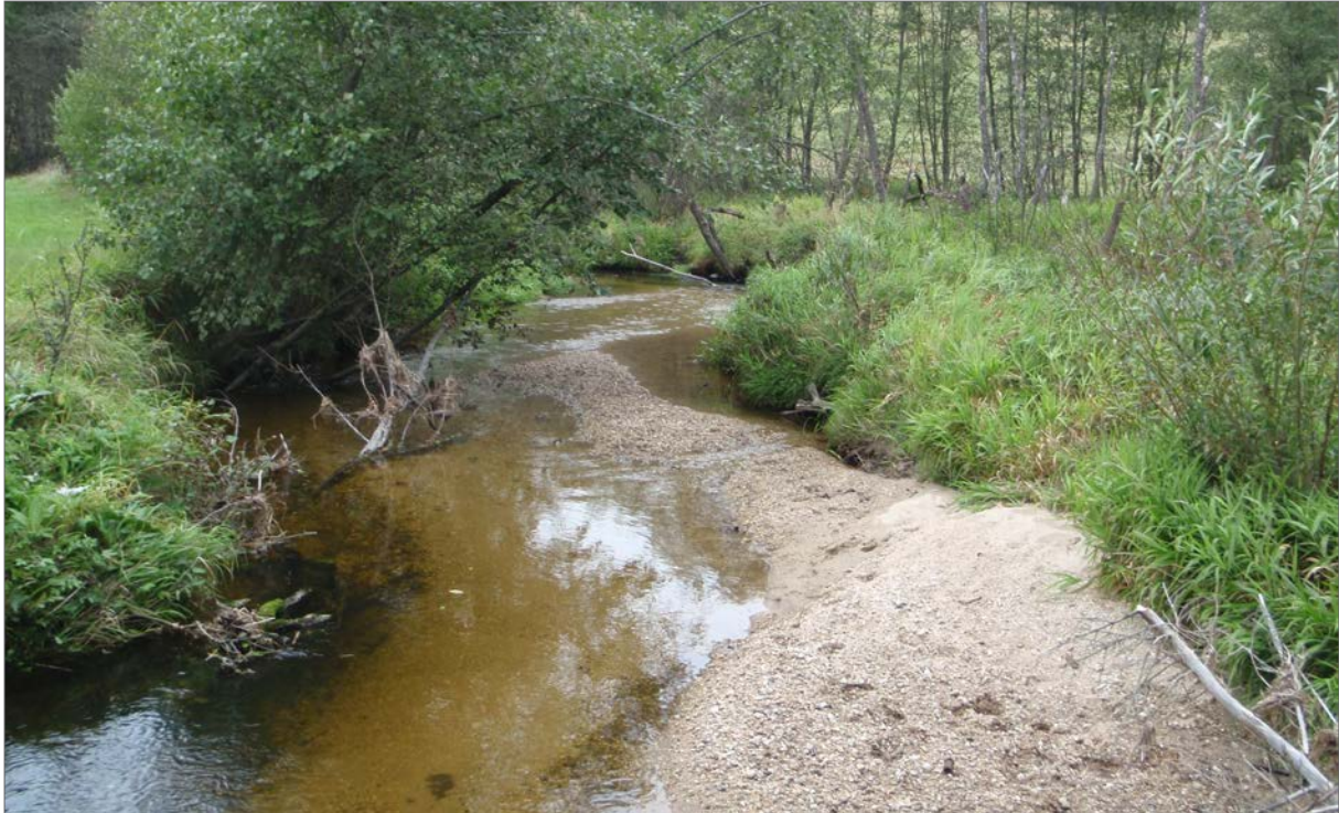
Fig. 165. Deterioration of the riverbed by sand deposits. Massive erosion from Kabelský potok stream and other sources in the catchment completely clogged the originally solid gravel bed of the Malše River.
