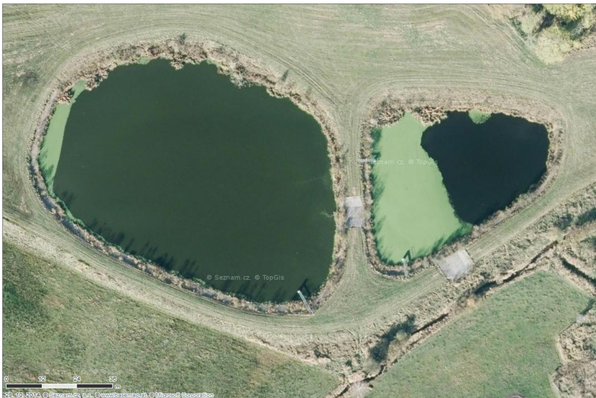
Fig. 111. Aerial view of low-loaded biological ponds for post-treatment in Zbytiny Source: Mapy.cz, © Seznam.cz, a. s., © TopGis, s. r. o.
