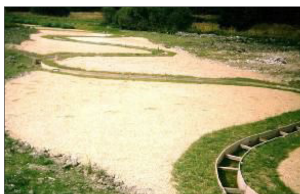
Fig. 173. LRRF – Lužní potok NNR – around the still dry channel, gradually rooting turf can be seen. The remaining areas of both RRFs (Fig. 172) will then be covered with pre-composted soil enriched with calcium in organic form (See Annex 4 for possible errors in construction).
