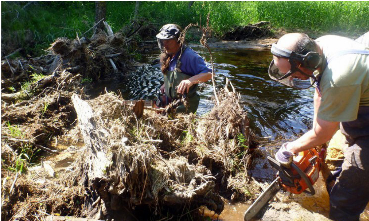
Fig. 207. Example of making watercourses passable. Removing an obstacle threatening a valuable meander above Spálenec RRF centre.
