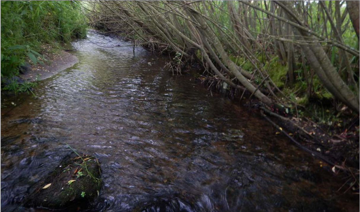
Fig. 200. Example of maintenance-free fascine bundles. Condition of fascine bundle after 10 years (800 m above sea level), clear flow profile, young trunks are growing upright.
