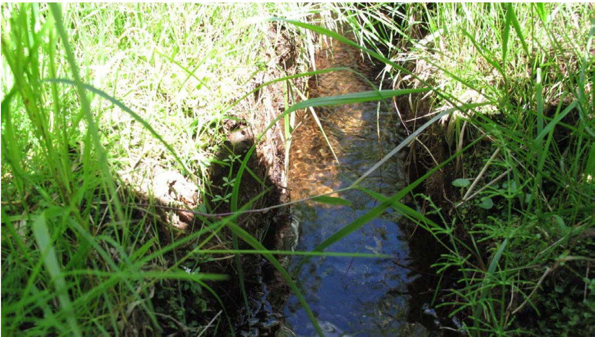
Fig. 219. Example of a food rill. Food rills should be checked regularly and restored to their original width every few years because they gradually become clogged and overgrown. Cleaned food rill in the Lužní potok stream catchment.
