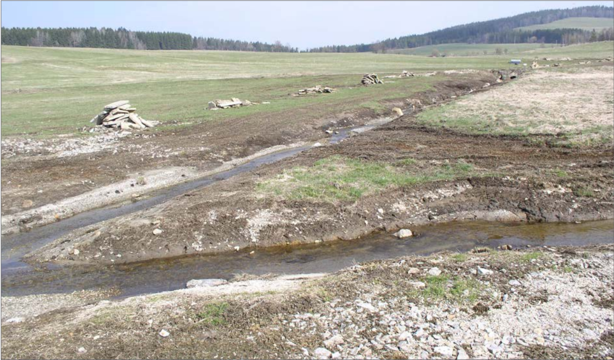
Fig. 167. Zbytinský potok stream and Sviňovická strouha stream (confluence) immediately after restoration. On the left side, next to the channel of the Zbytinský potok stream, the remains of the concrete bank protection of Sviňovická strouha stream are visible on piles; the Sviňovická strouha stream remained deep and straight.
