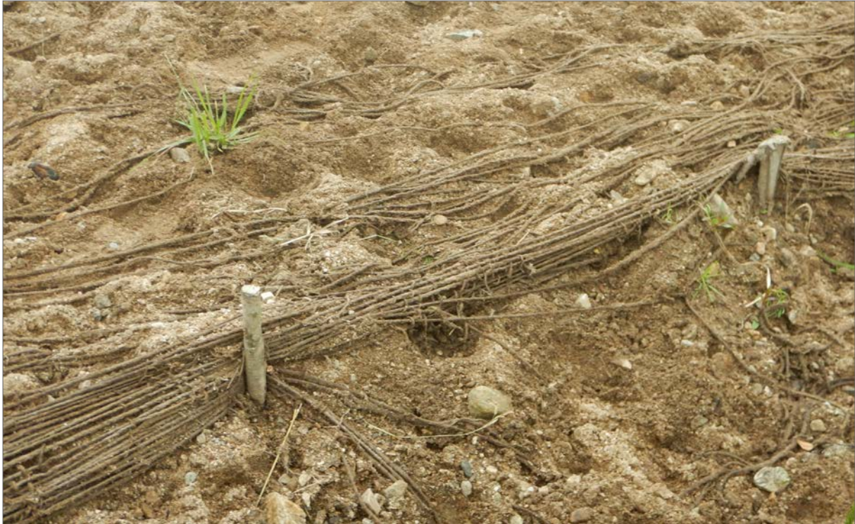
Fig. 212. At present, the meander is generally stable, although most willow cuttings have not taken hold.
