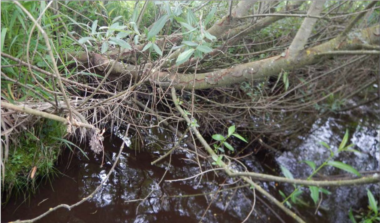
Fig. 202. Example of maintenance-free fascine bundles. The horizontal trunks reaching into the flow profile must be cut.
