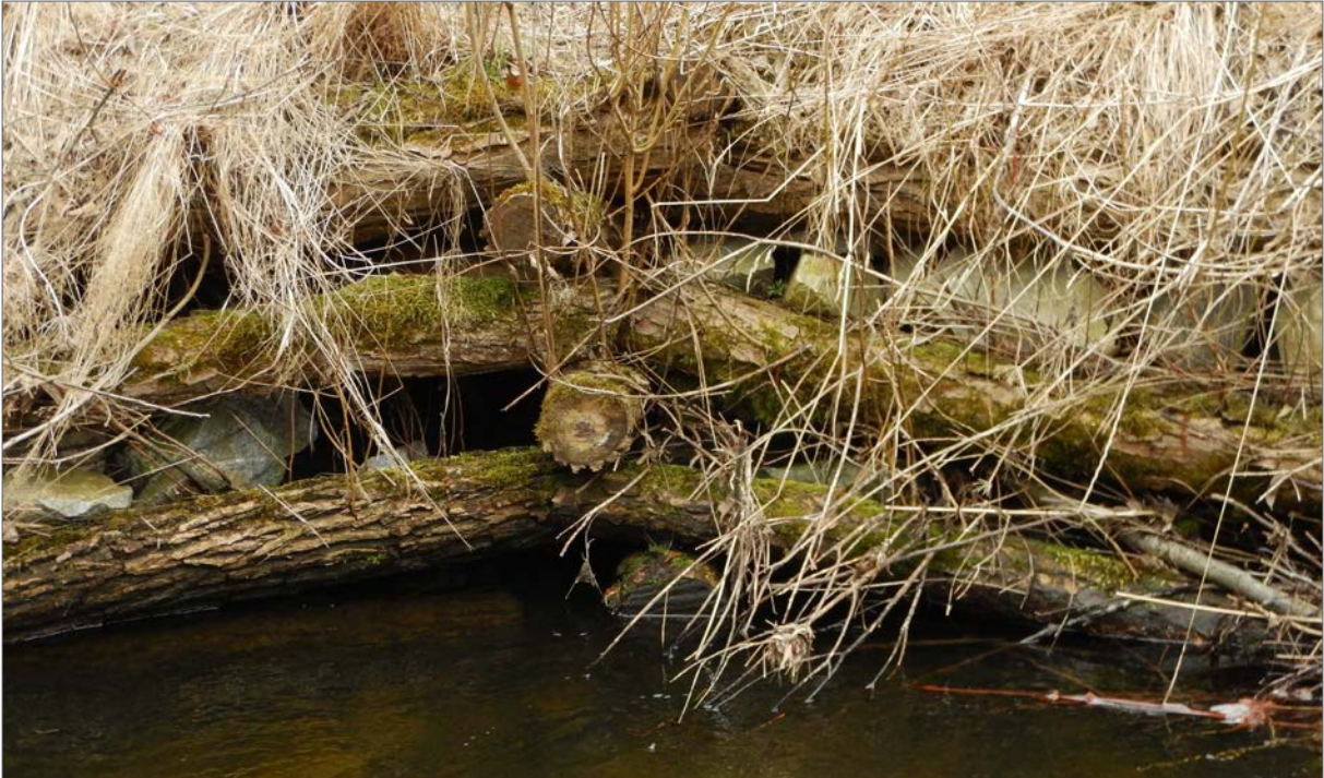
Fig. 204. Living willow log structures. Close-up view of a growing willow log structure in early spring-time – willow trunks interspersed with quarry stone.
