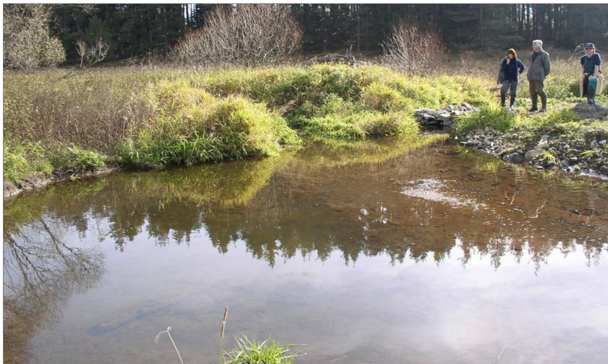
Fig. 186. Restoration modifications above the mouth of Zbytinský potok stream where it enters the Blanice River. Large sedimentation pool at Zbytinský potok stream in 2005.
